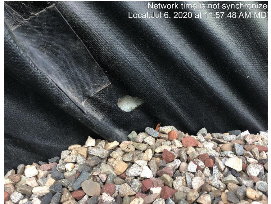
Photo #1455 Multiple holes in tank containment liner.
