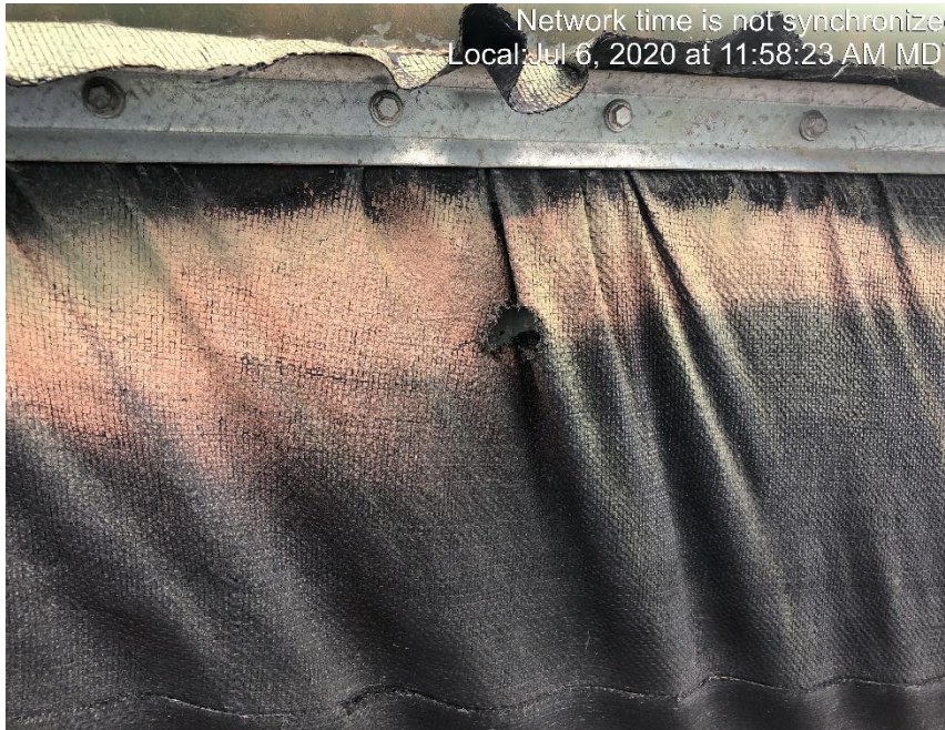
Photo #1456 Multiple holes in tank containment liner.
