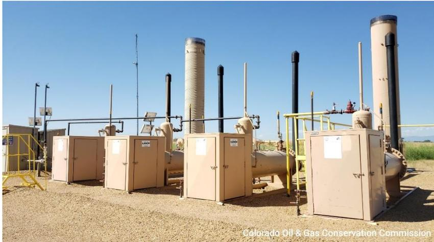
**Photo 13 Horizontal Heated Separators and ECDs.**
