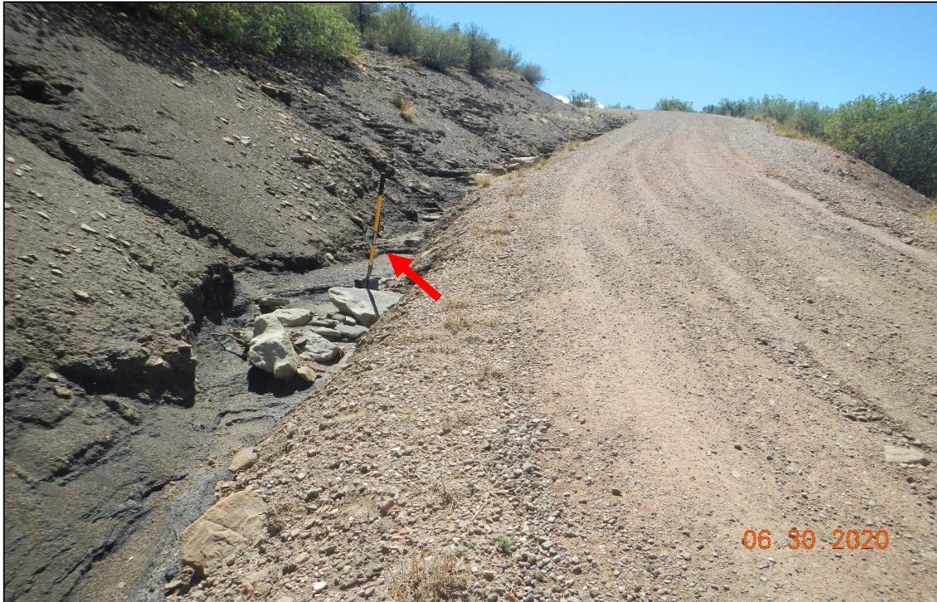
Photo 1. Facing southeast along the access road. There is erosion occurring along the side of the road and there are no BMP's In this area along the road.
