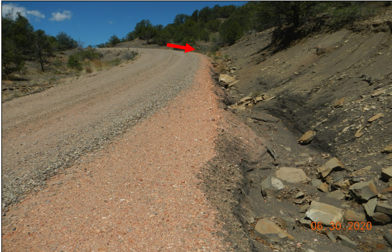
Photo 6. Facing back toward the west. There is a long stretch of road (from red arrow) which does not have BMP's which is contributing to the volume of stormwater directed down the side of the road.
