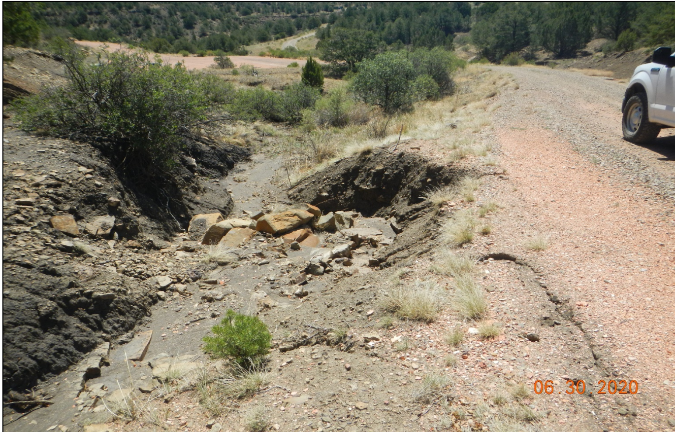
Photo 5. Facing southeast along the access road. Stormwater diverted along the road is causing erosion in this area.
