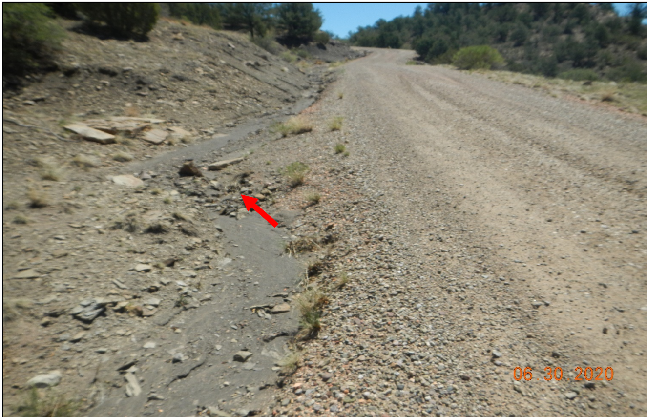
Photo 3. There is a culvert at this point along the road which has filled in with sediment.
