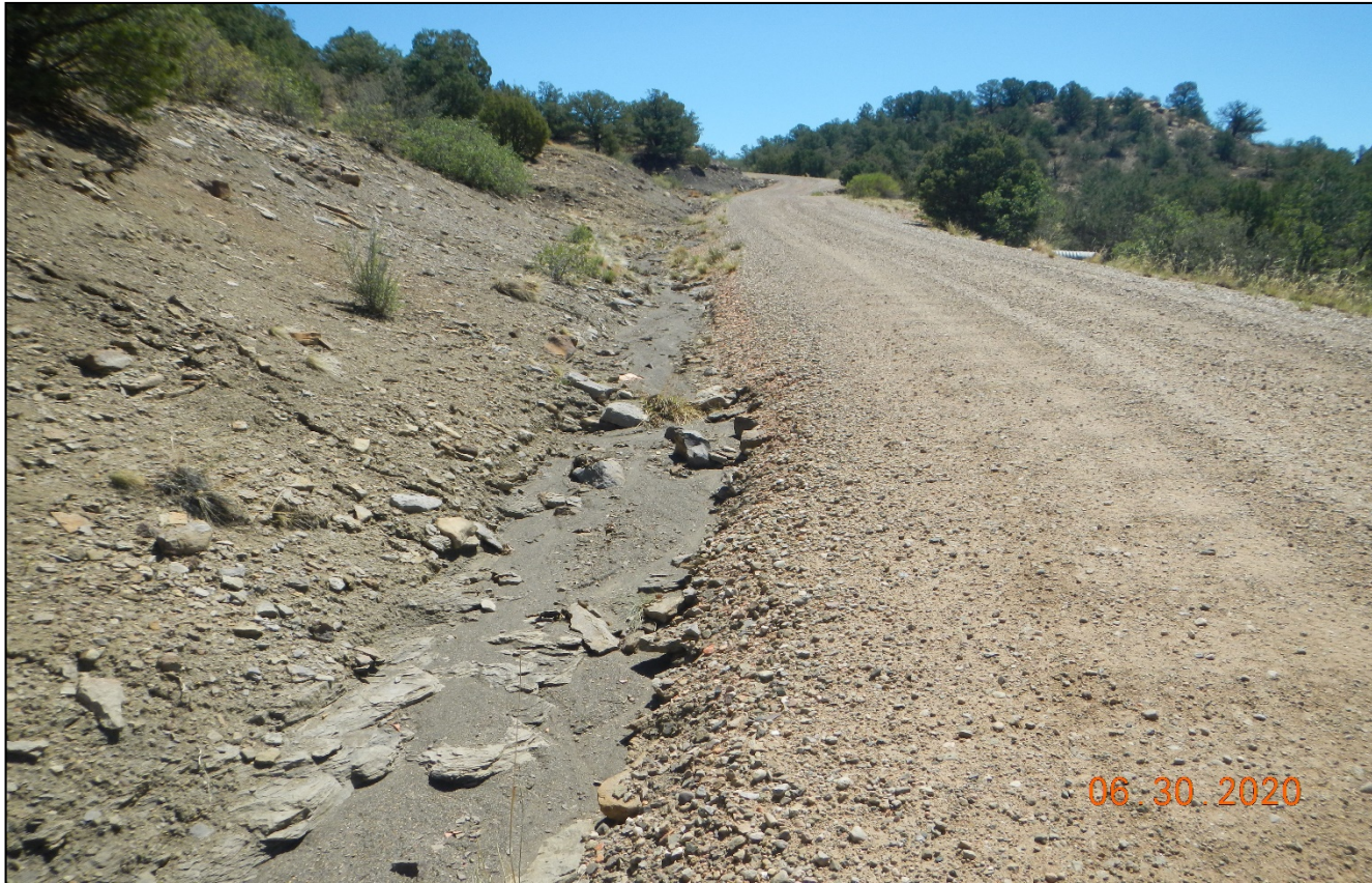
Photo 2. Facing east along the road. There is a long stretch of road which does not have culverts or BMP's which is contributing to the volume of stormwater directed down the side of the road.
