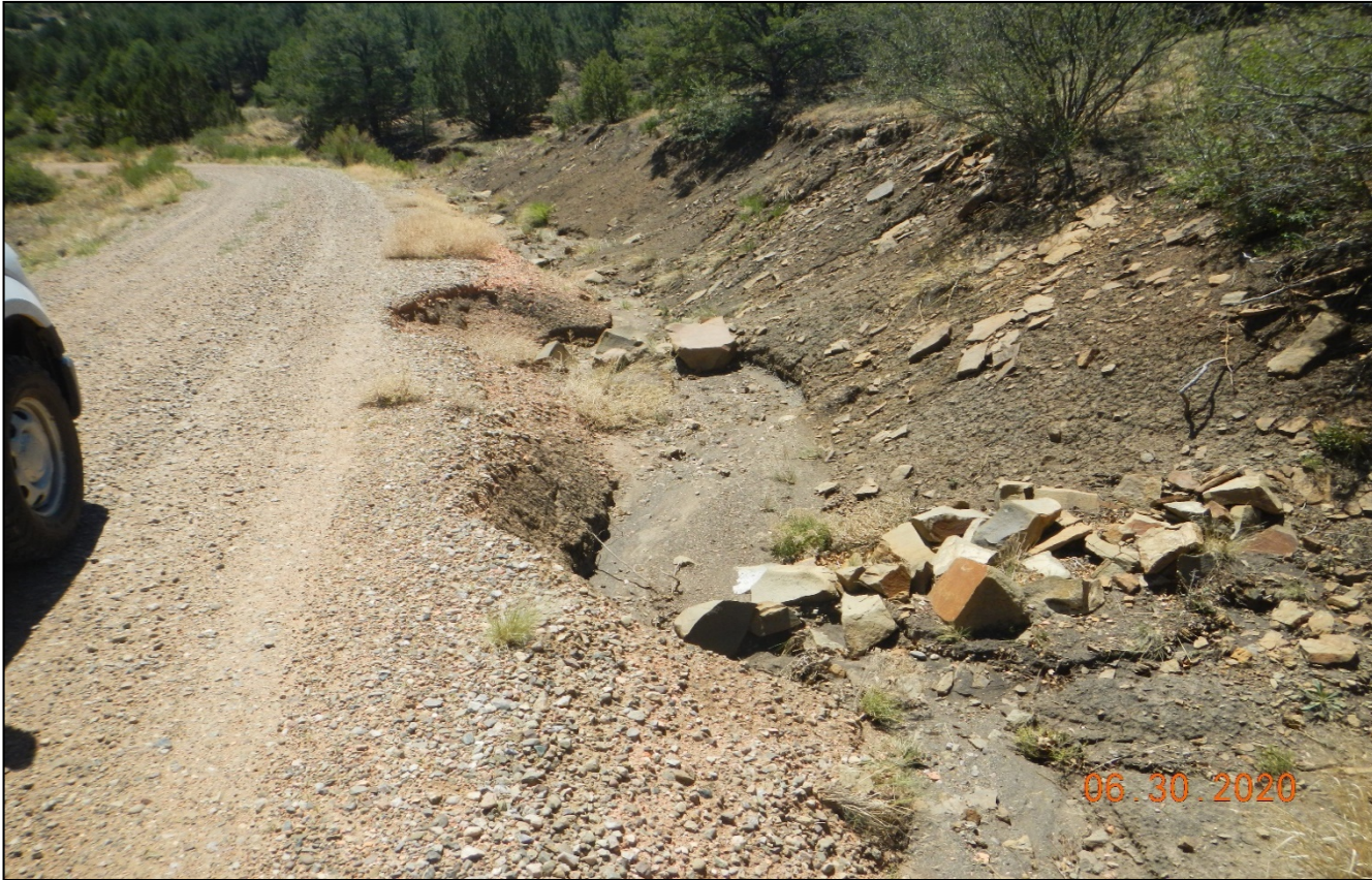
Photo 7. Facing southeast along the opposite side of the road. Rock check damns have failed in this area.
