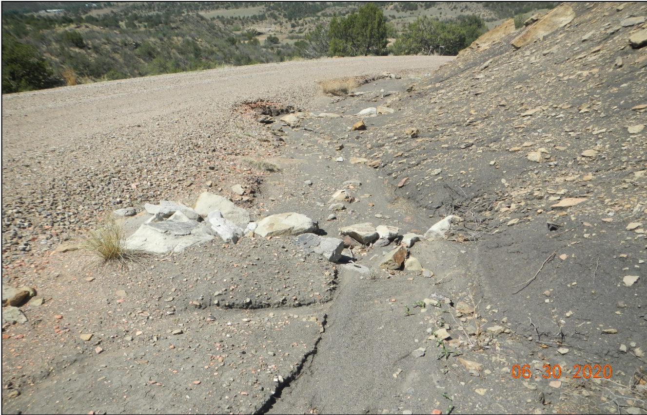
Photo 4. Facing back toward the southwest near the top of the hill toward the location. These rock checkdamns have filled in with sediment and are displaced.
