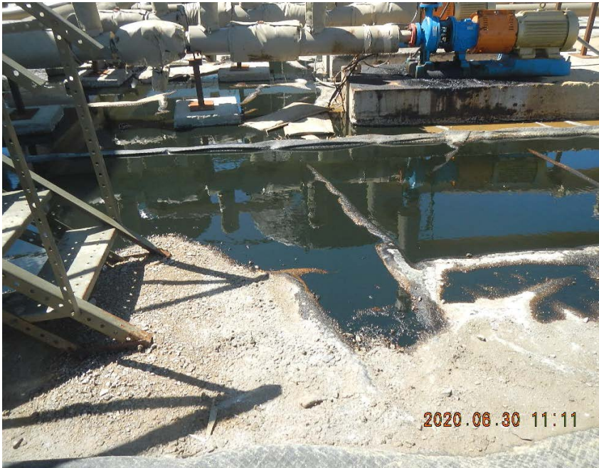
Oil pooling on liner.
