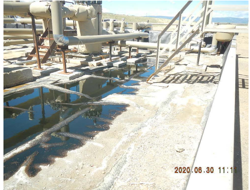
Salt staining on liner throughout secondary containment.
