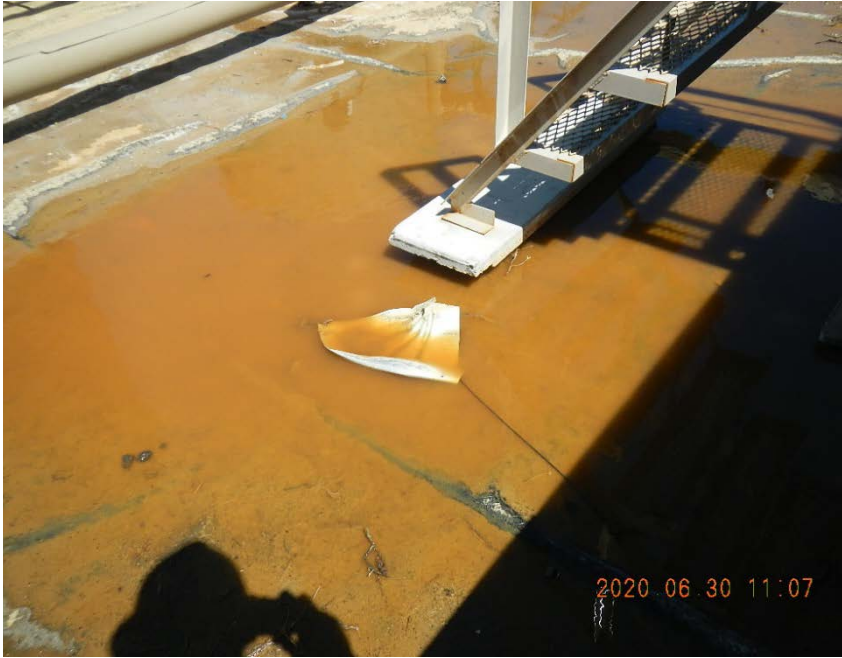
Pipe and stair supports deteriorating, metal sheeting on liner.
