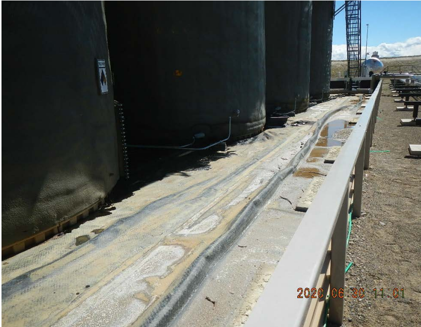
Concrete weight/anchor with rebar (trash/debris) with potential to puncture or compromise liner.
