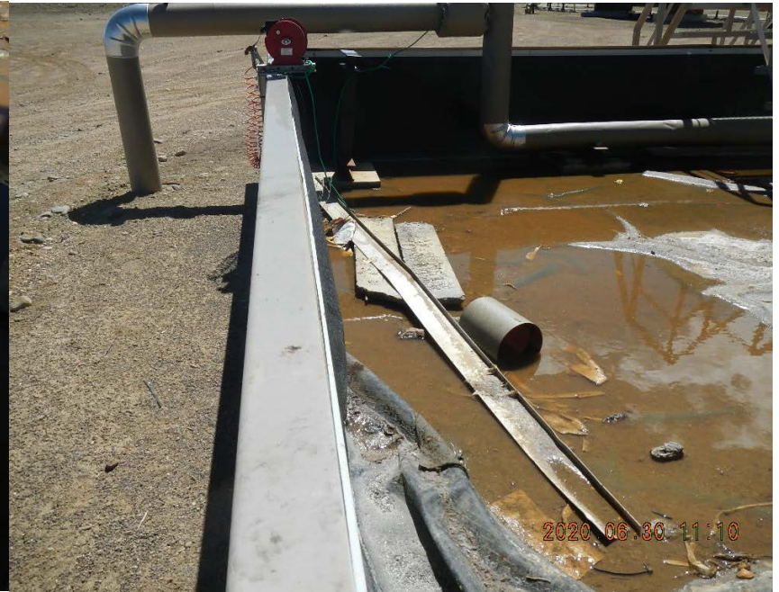
Trash/debris metal sheeting on liner. Note the folds in liner.
