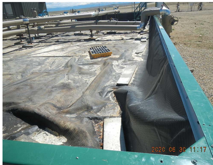
Concrete weight/anchor with other debris on liner with the potential to puncture or compromise liner. Note how liner is wind blown with folds.
