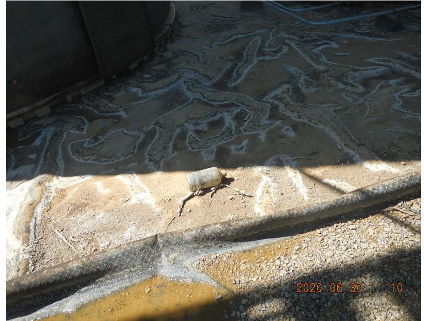
Trash and folds in liner.
