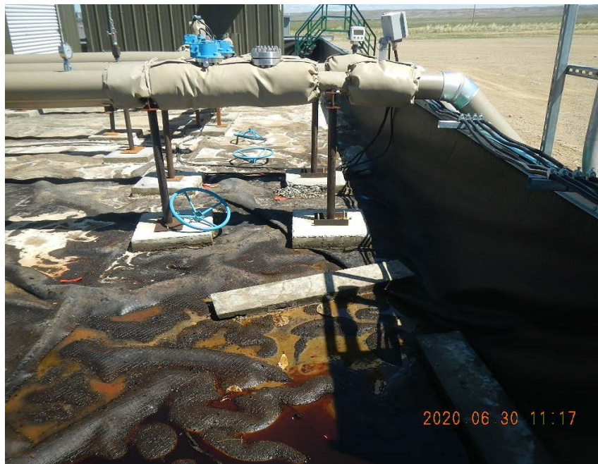
Concrete weight/anchor with rebar and valve handles with potential to puncture or compromise liner. Oil pooling on liner.
