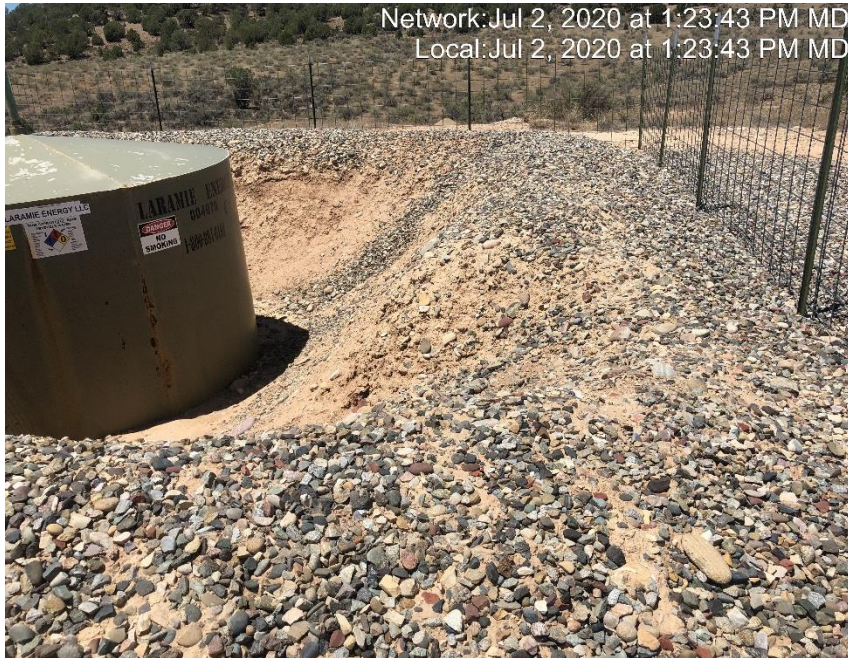
Photo #1451 Secondary containment berm has eroded.
