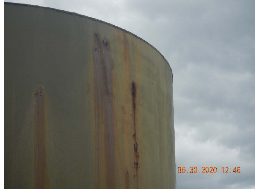
Photo 2. Holes in tank.
