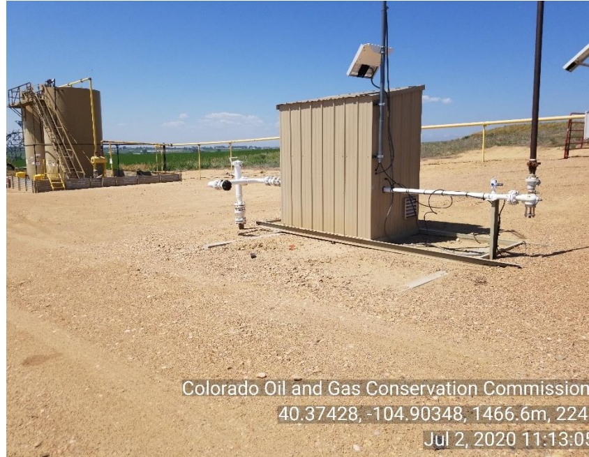
Photo 3: Gas meter removed
