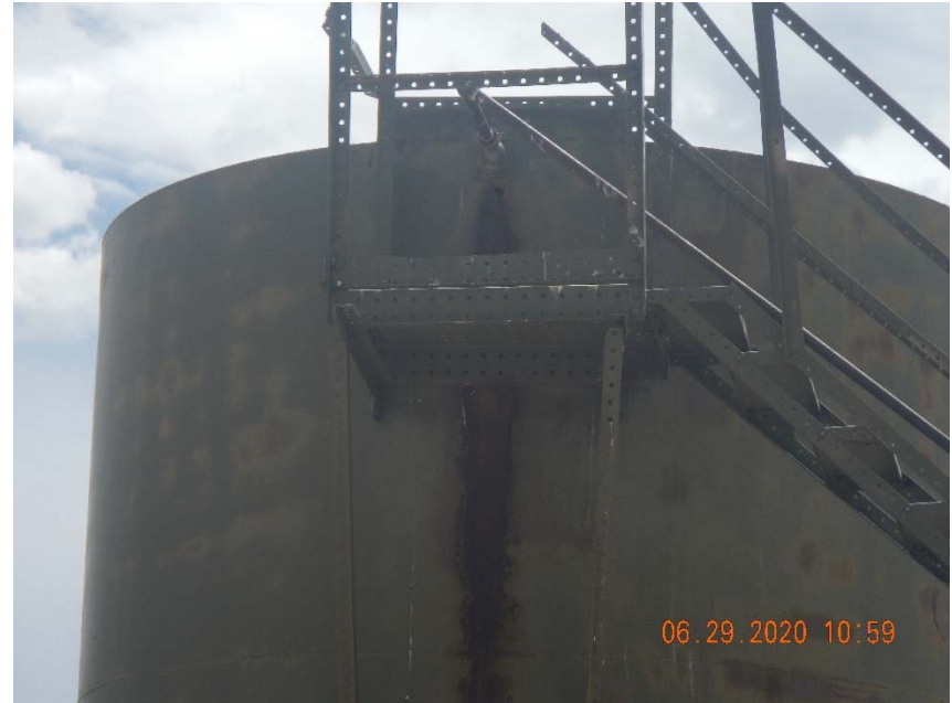
Photo 3. Hole in tank.
