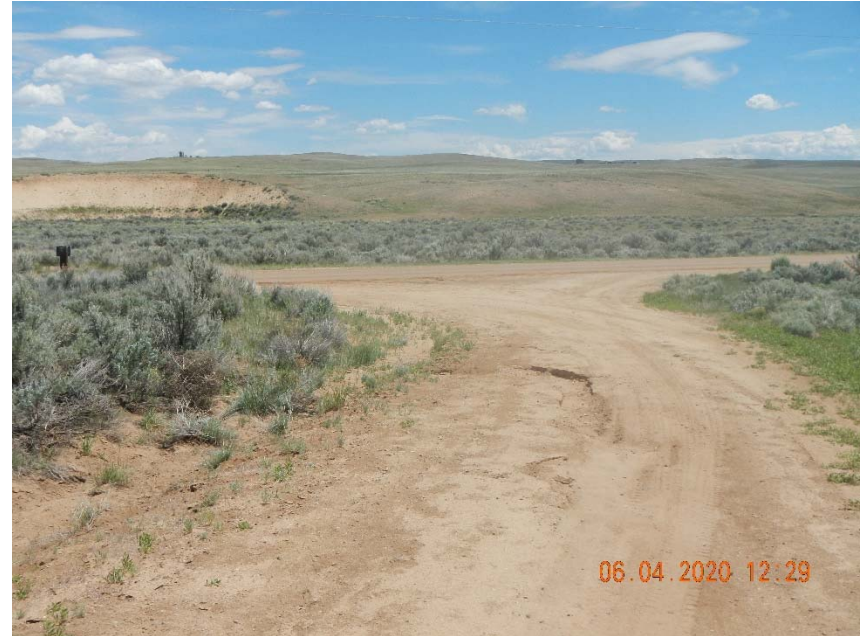
Photo 4. Example of sediment migration on access road.
