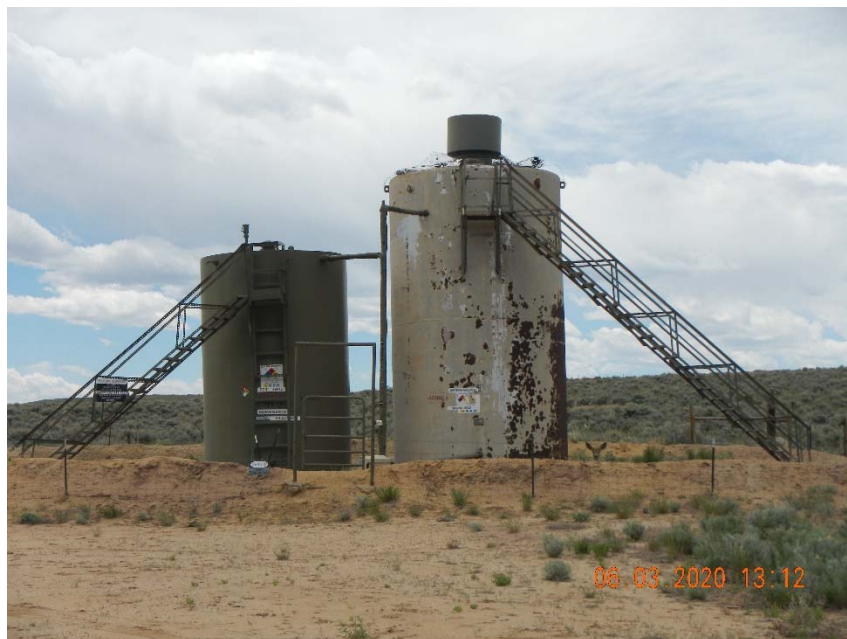
Photo 2. Tank top insulation on 400 BBL tank peeling off.
