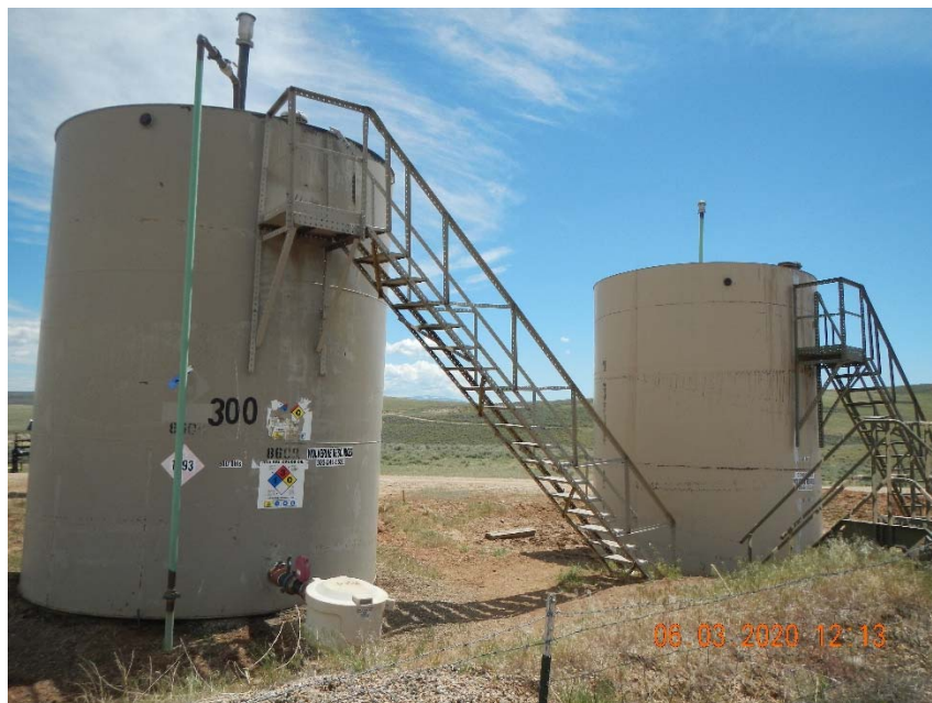
Photo 2. Incomplete tank labels.
