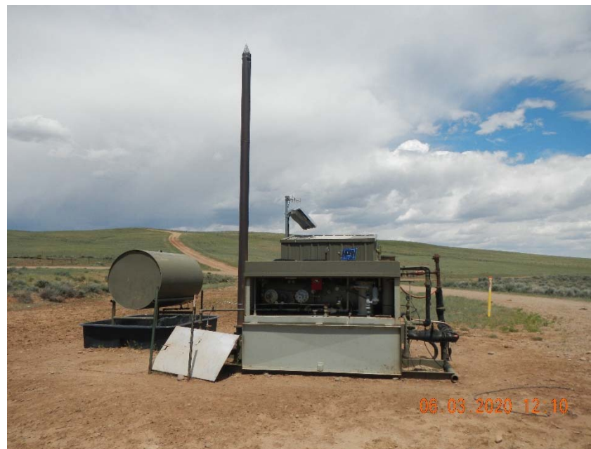
Photo 3. Separator does not appear operable.
