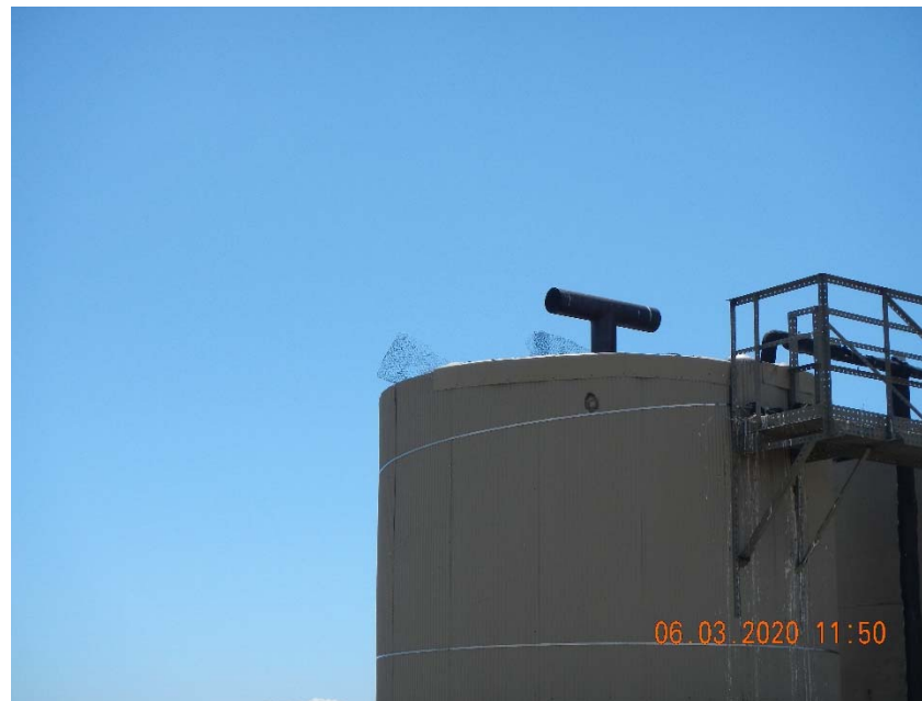
Photo 3. Tank top insulation peeling off.
