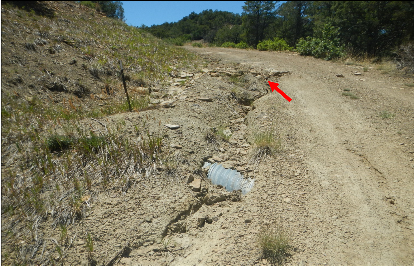
Photo 4. There is erosion occurring down the road and stormwater is not properly diverted toward the culvert in this area.
