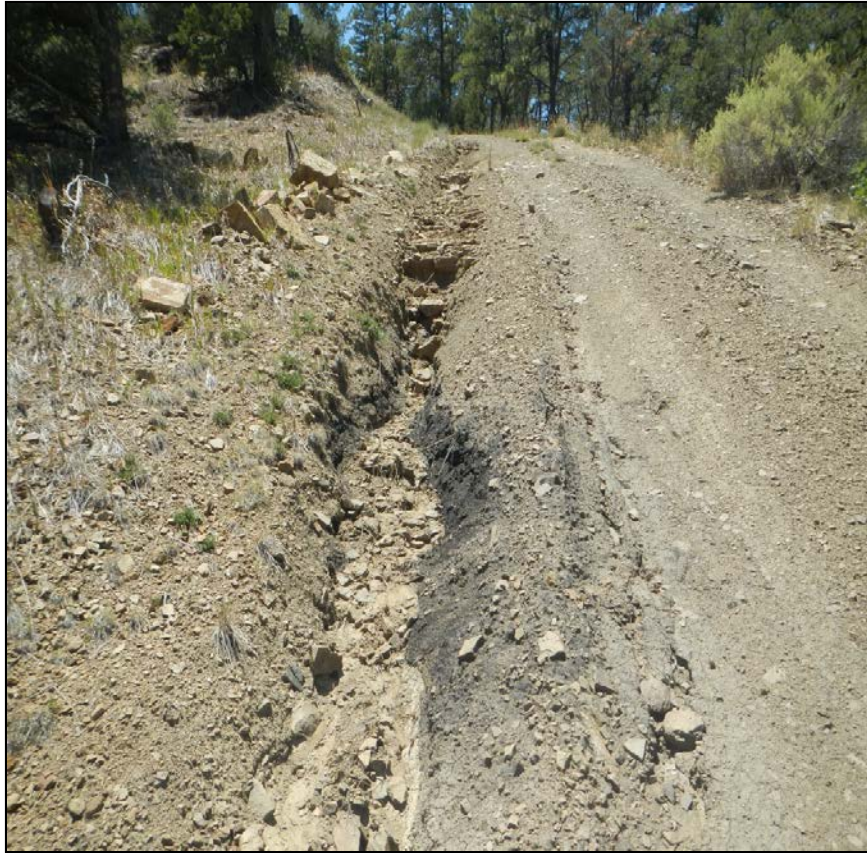
Photo 5. Facing west along the road near the top of the hill. There is an erosion channel that has formed in this area.
