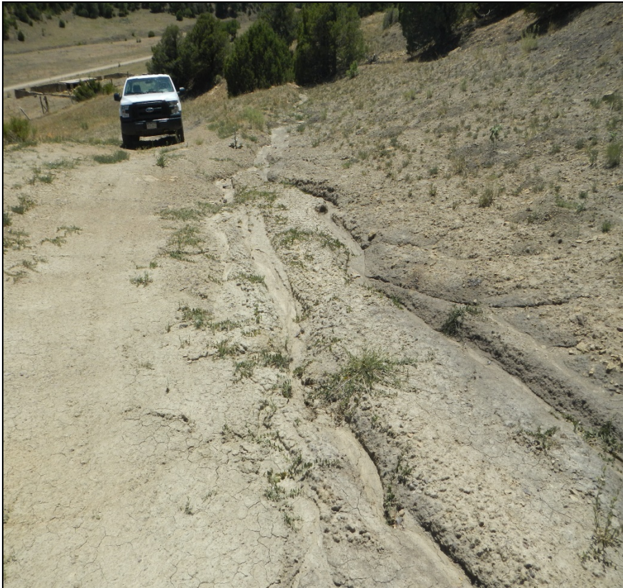
Photo 1. Facing south near the beginning of the access road. The water bar installed is diverting stormwater off the road however, erosion channels have developed.
