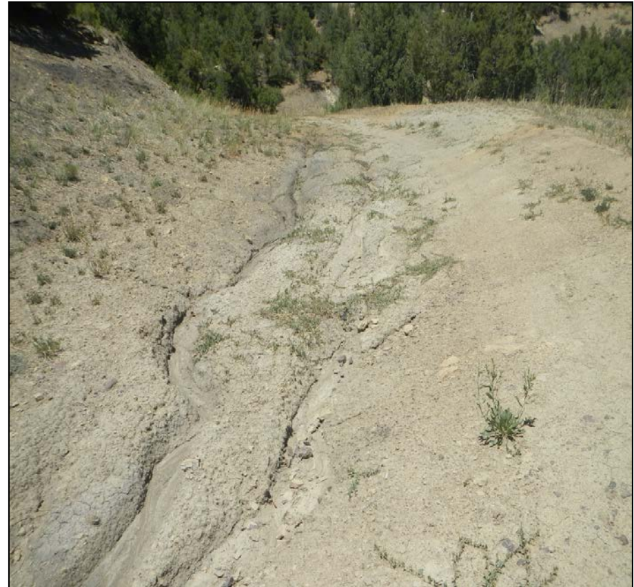
Photo 2. Facing back to the north. There are erosion channels near the water bar shown in previous photo.
