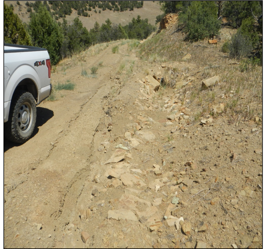
Photo 6. Facing back toward the east near the top of the hill shown in area of previous photo. Stormwater is not fully being divert toward the culvert at this point.
