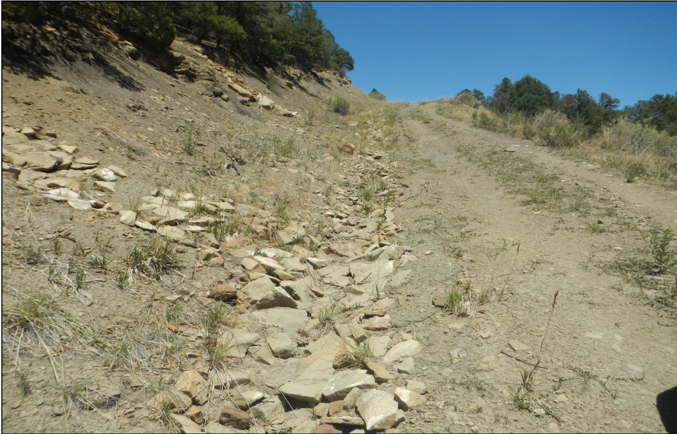
Photo 3. Facing northeast along the road ascending the hillside. Rip/rap is installed along the side of the road to prevent erosion.
