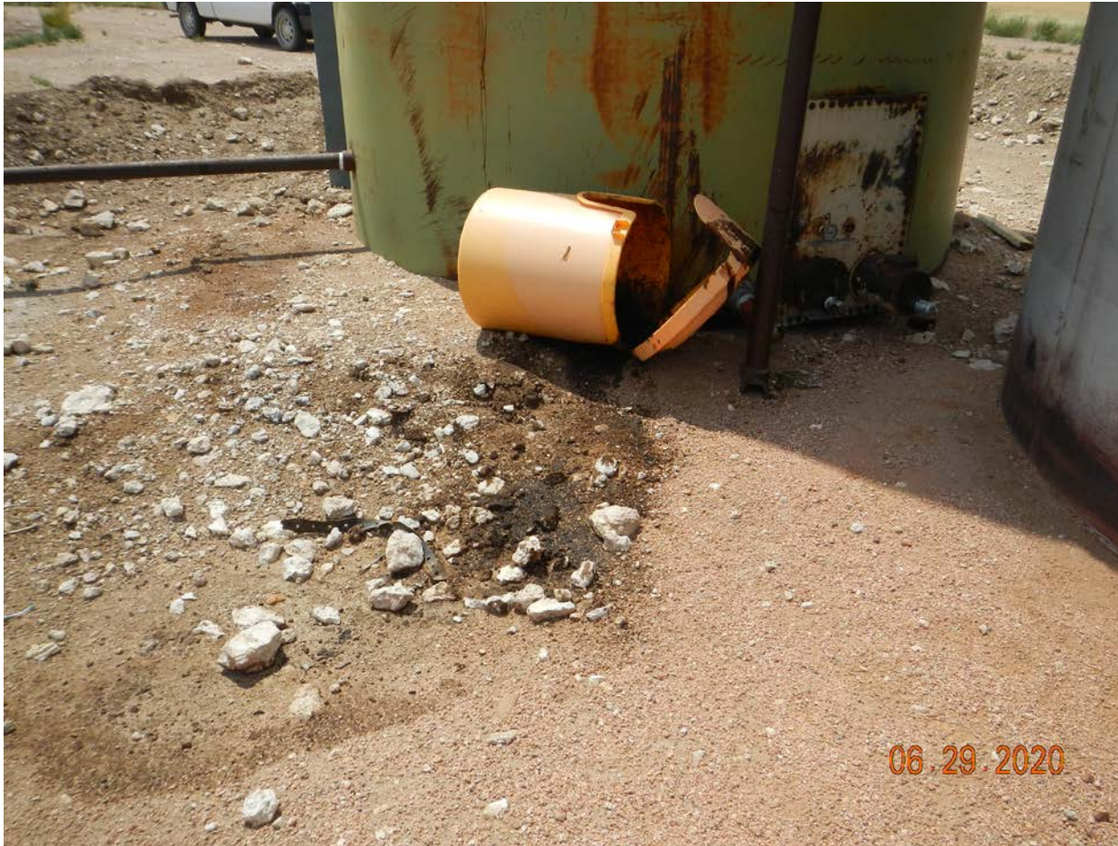
Photo # 4 – South side of tank battery. Yellow containment bucket on its side, oil stained soil
