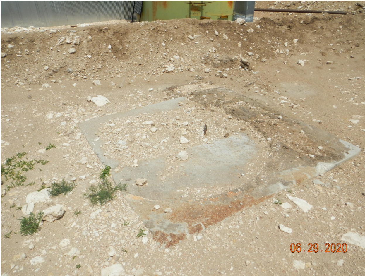
Photo # 7 – West side of tank battery former separator concrete foundation requires removal and disposal
