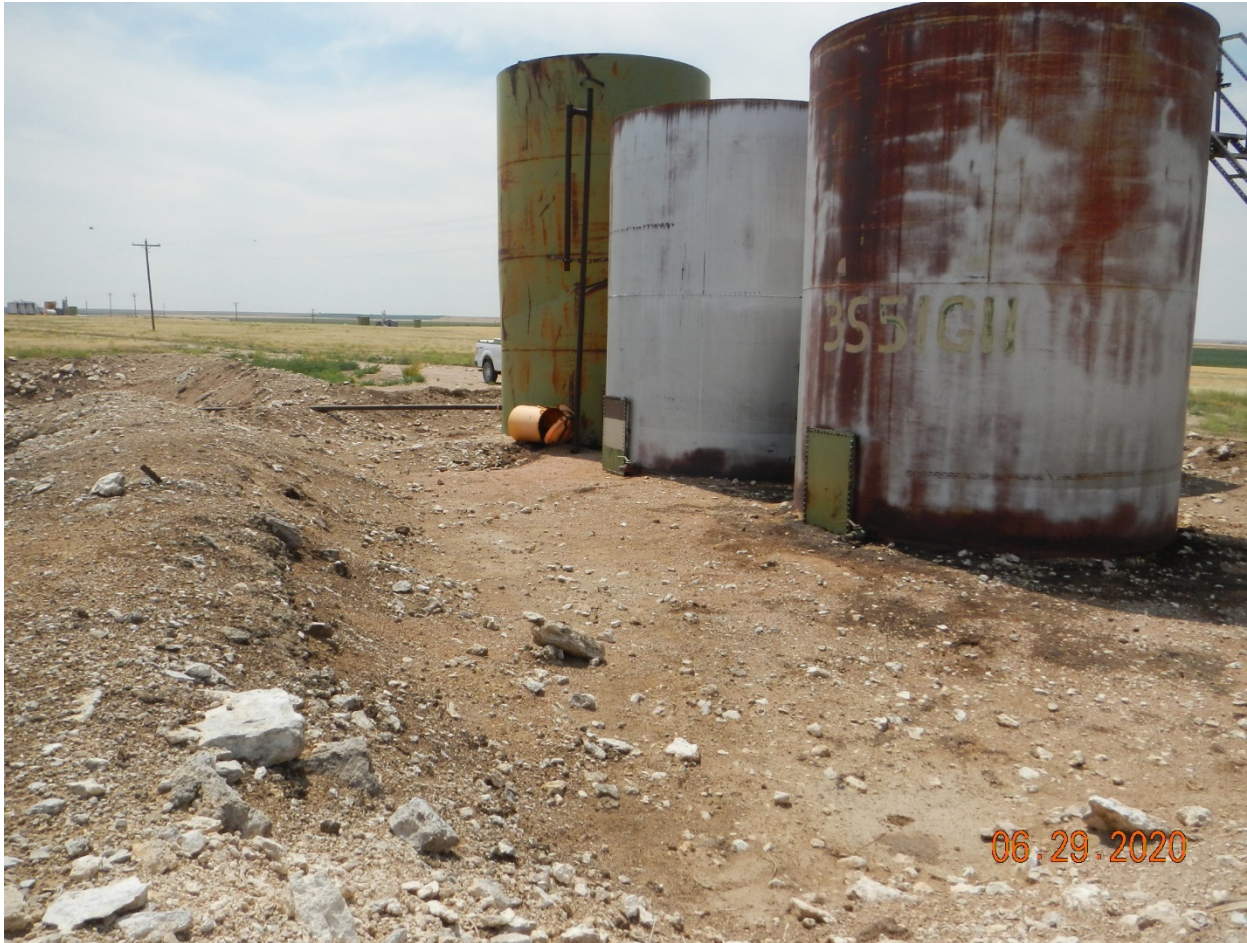
Photo # 3 – South side of tank battery. Yellow containment bucket on its side, stained soil on east side of battery
