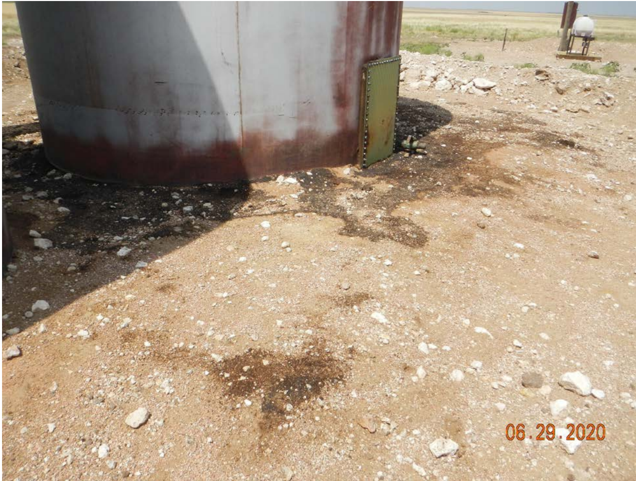
Photo # 5 – South side of tank battery oil stained soil around produced water tank
