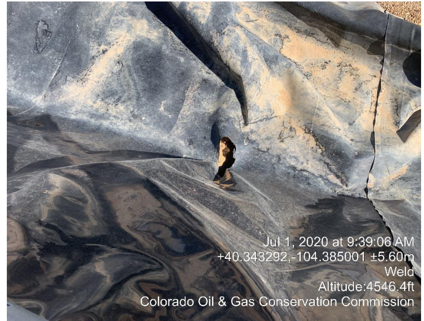
Photo #8 Hole in liner
