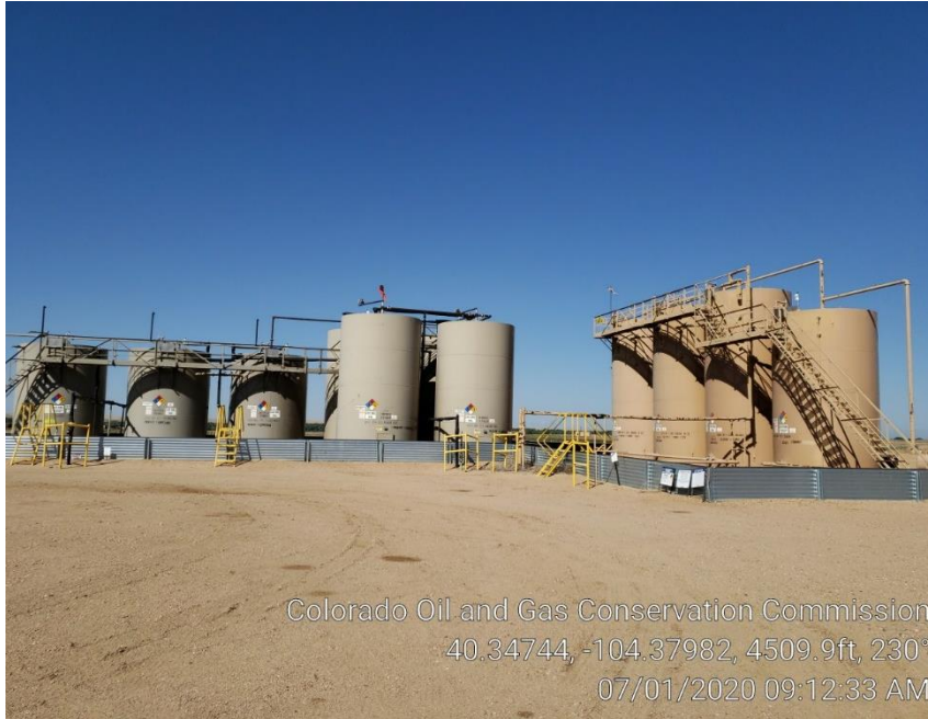
Photo #1 Tank Battery
