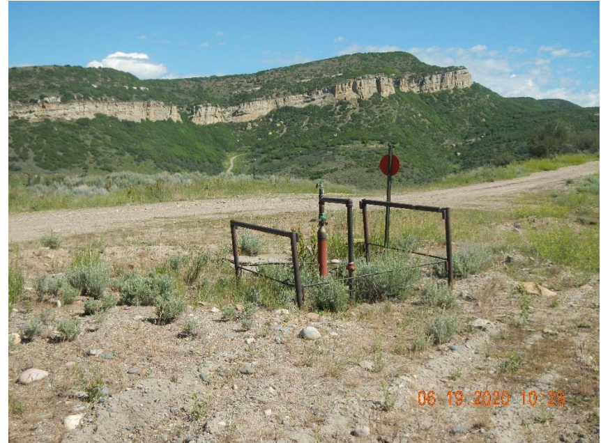
Photo 3. 2 -2" steel risers not marked for abandonment or LOTO.
