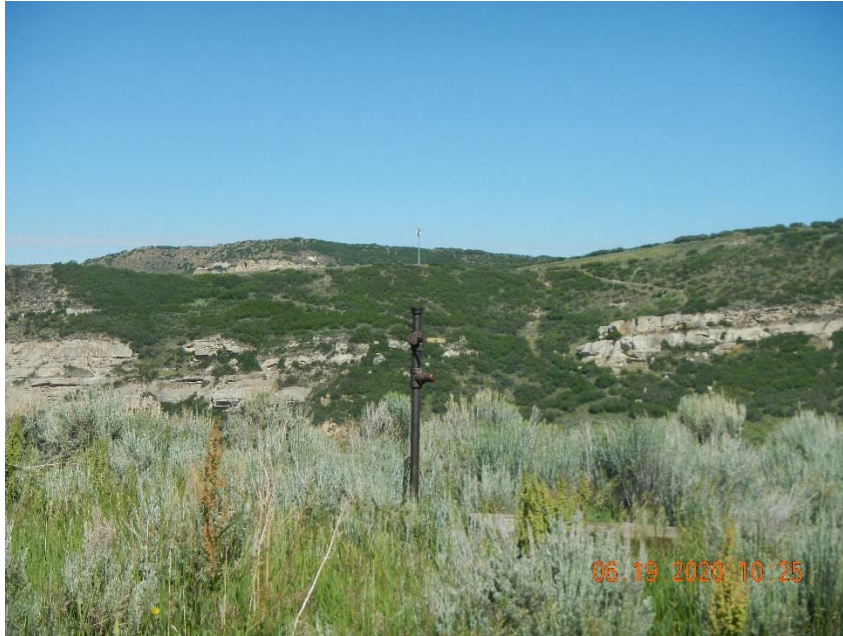
Photo 2. 1 – 2" steel riser not marked for abandonment or LOTO.
