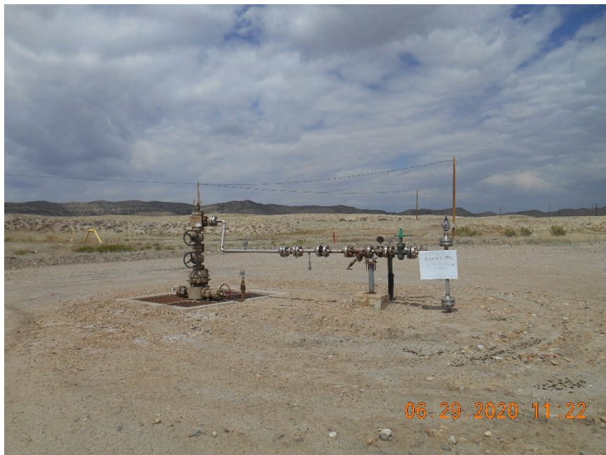
Injection wellhead. Sign installed. CA completed.
