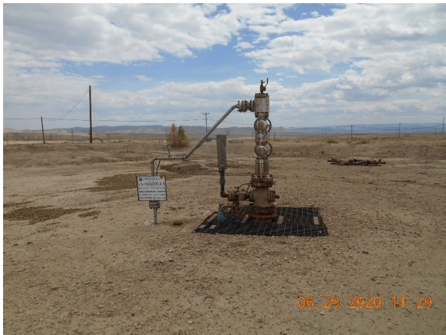
Injection wellhead. Sign installed. CA completed.
