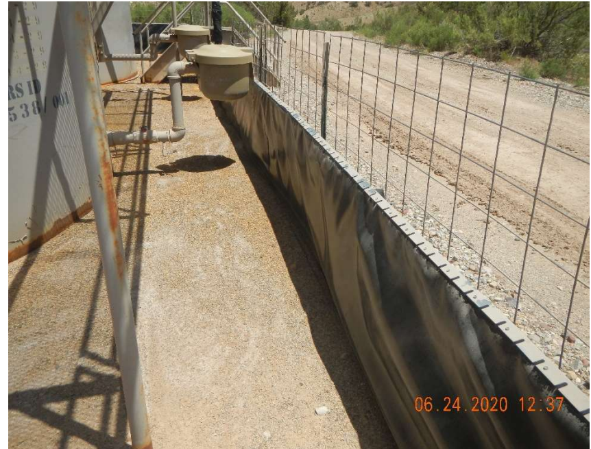
Tank battery secondary containment
