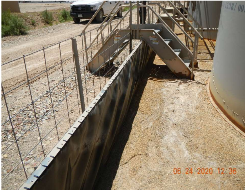
Tank battery secondary containment
