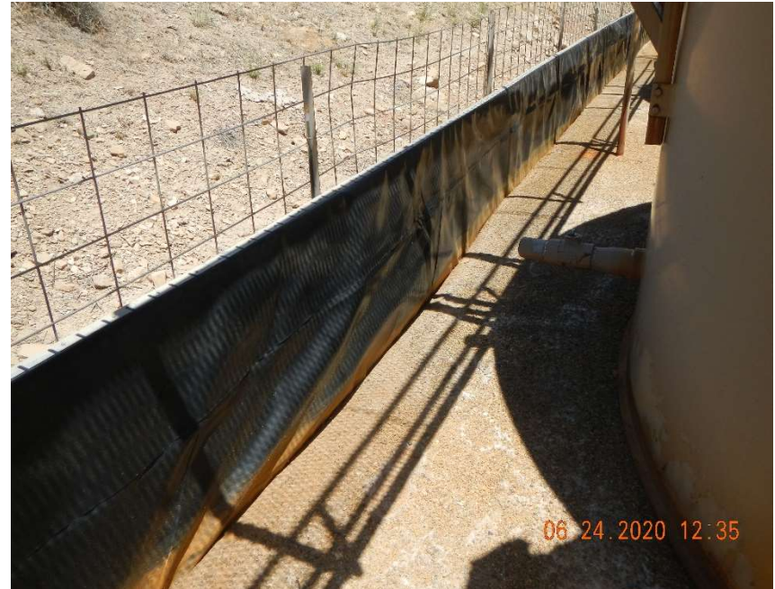
Tank battery secondary containment liner and residual staining ring
