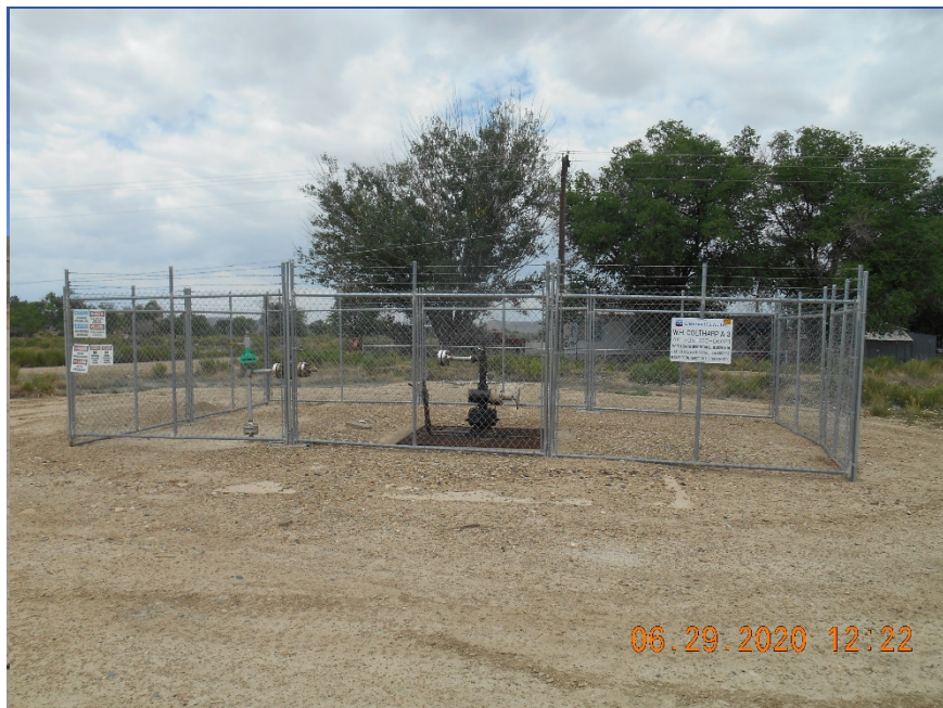
Injection wellhead. Temporarily Abandoned
