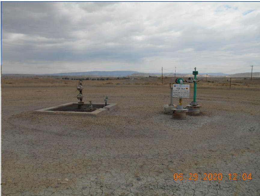
Injection wellhead. Temporarily Abandoned
