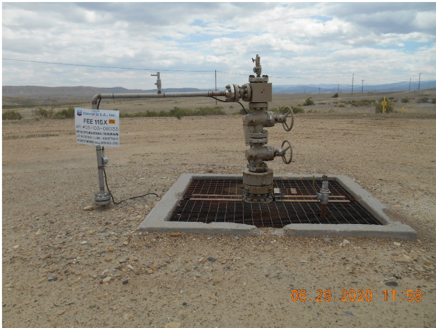
Injection wellhead
