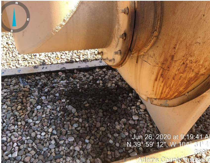
Photo #7 stained soil under separator and missing chunk if gasket in separator fire box.
