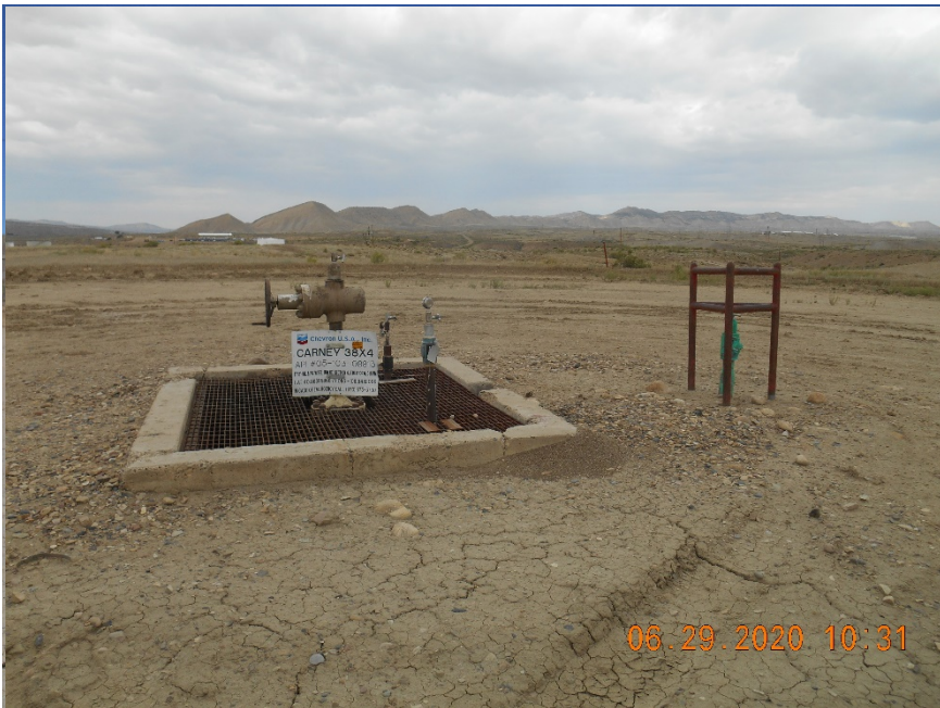
Injection wellhead. Temporarily Abandoned
