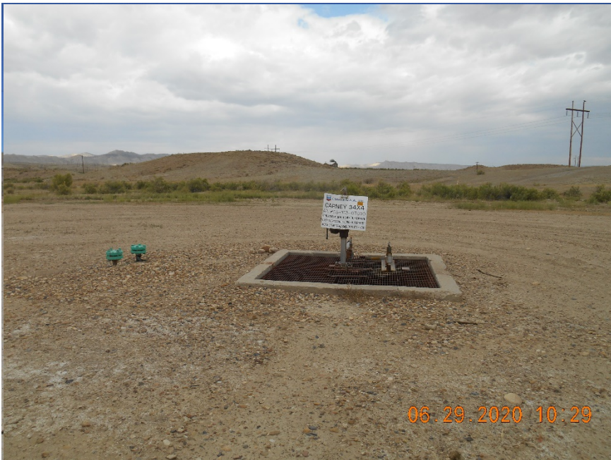
Injection wellhead. Temporarily Abandoned
