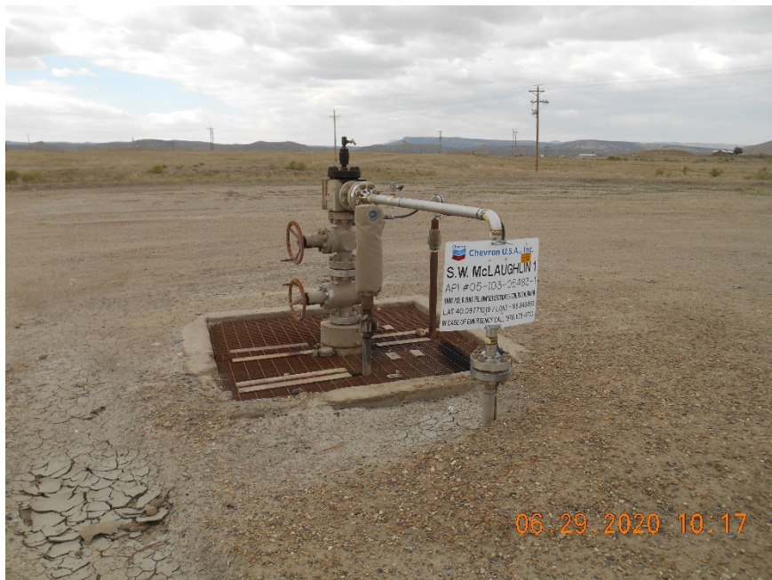
Injection wellhead
