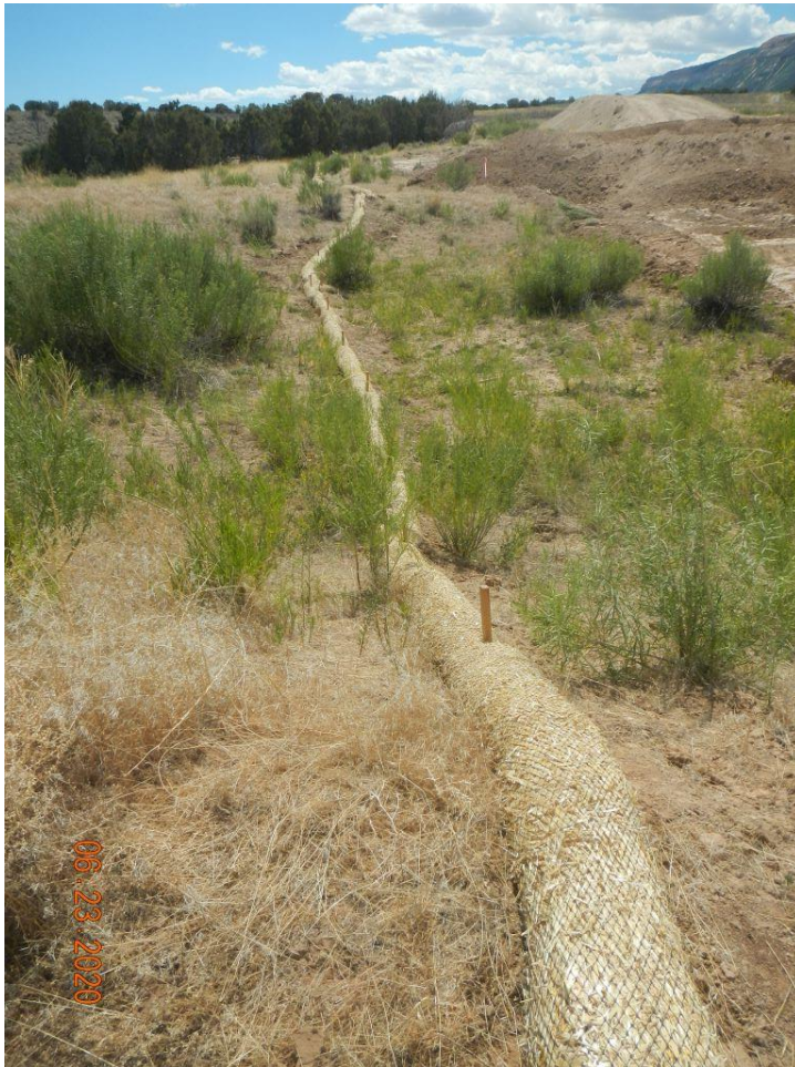
Photo#3: Wattles installed as perimeter control.
