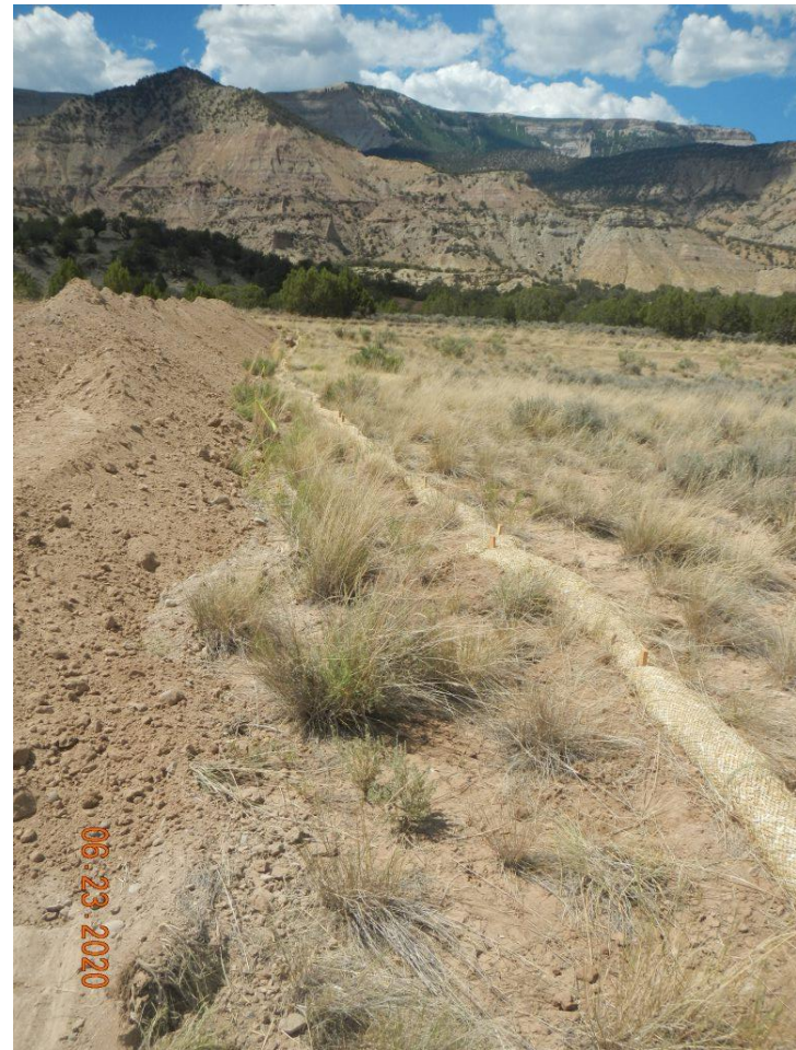
Photo#4: Wattles installed as perimeter control
