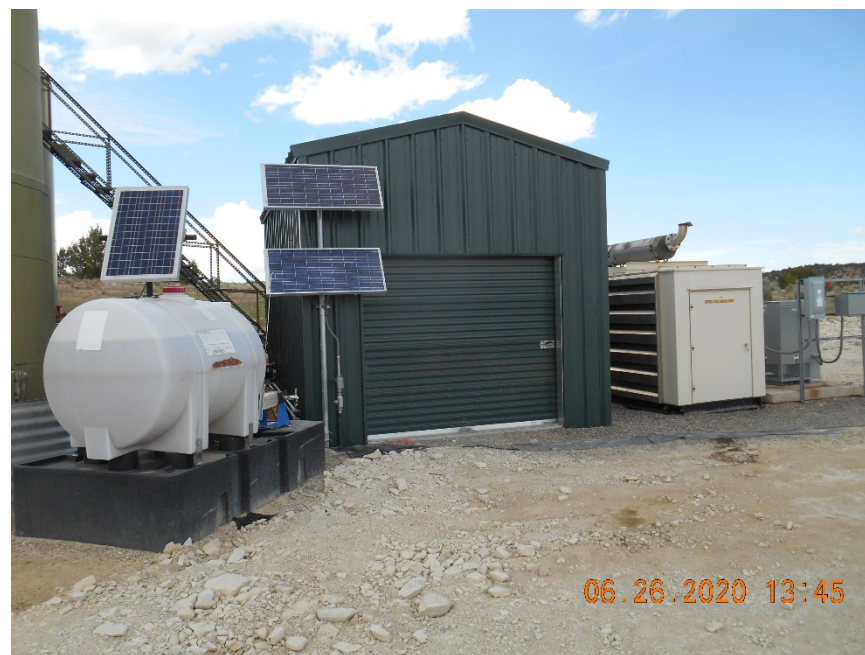
Pump Housing. Chemical injector with secondary containment. Generator
