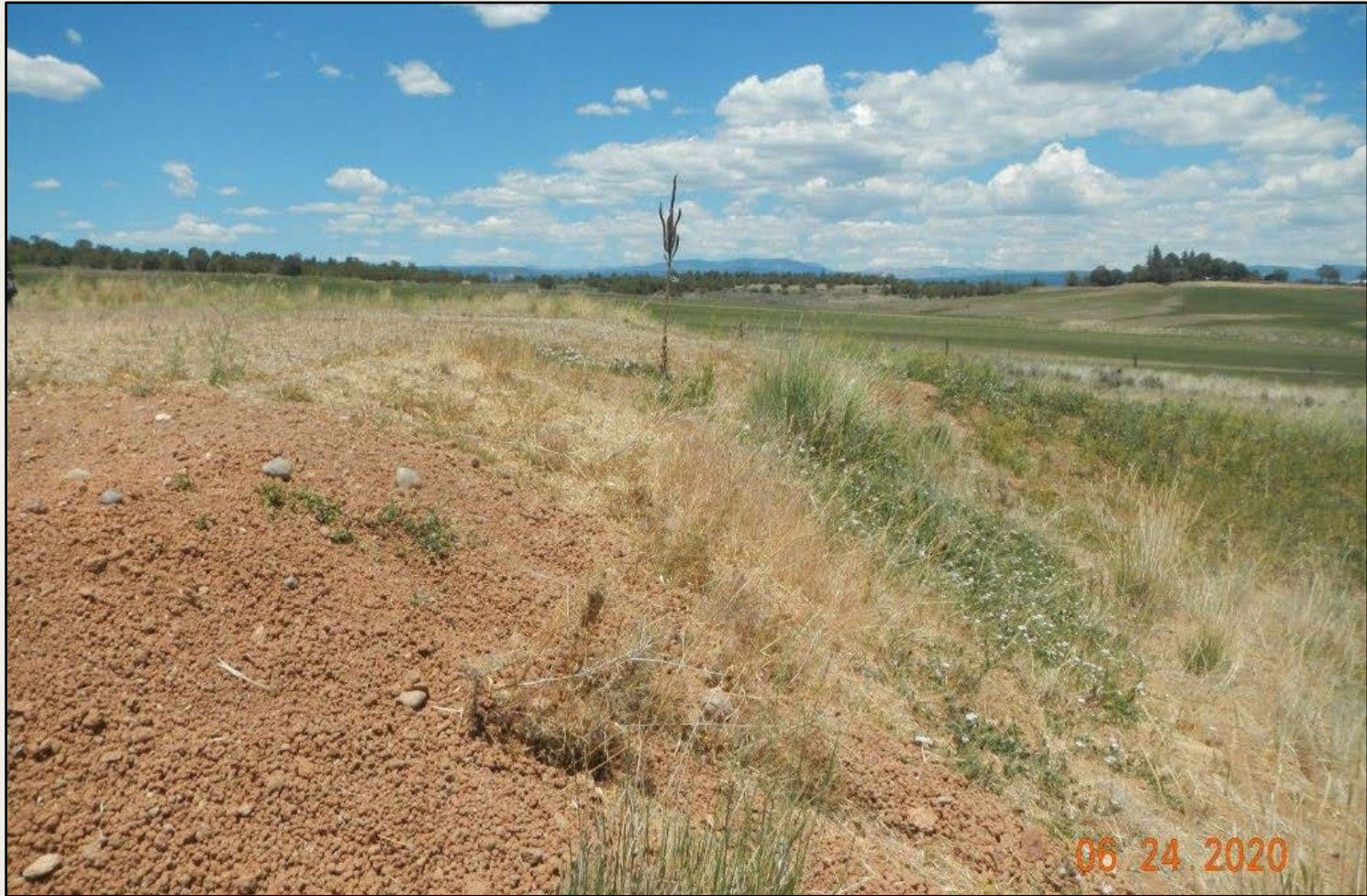
Photo 2. View of the eastern fill slope from the southeastern corner facing northward. Revegetation is progressing within portions of the interim reclamation area with crested wheatgrass, intermediate wheatgrass, and western wheatgrass, but remains sparse in portions and needs to be monitored.
