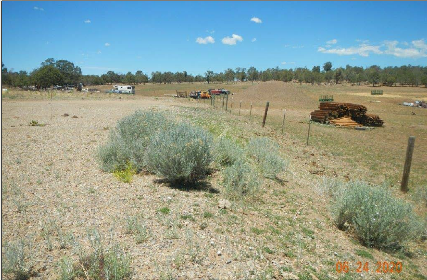
Photo 2. View of the northern fill slope from the southeastern corner facing westward. Revegetation is progressing, although grazed, with grasses such as crested wheatgrass and shrubby rubber rabbitbrush.
