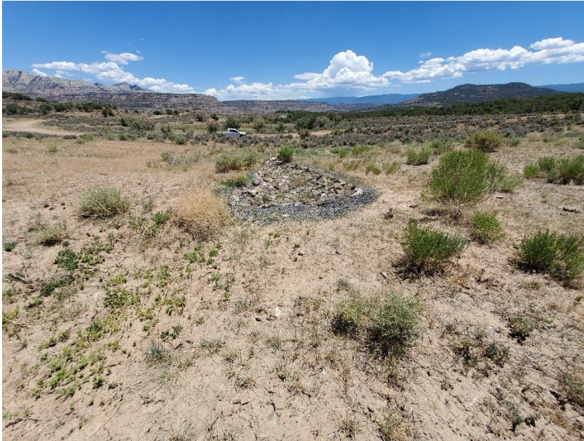
Photo 5: Photo taken from the east end of the Location, facing east. Photo shows an armored outlet on the Location. BMP appears to be in proper functioning condition.
