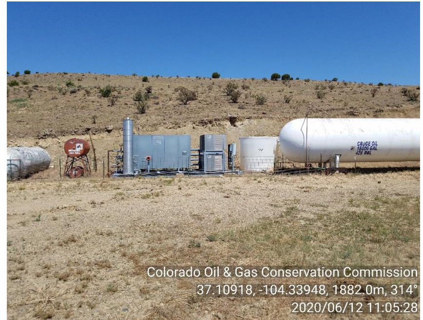
PHOTO 2: TANK BATTERY
