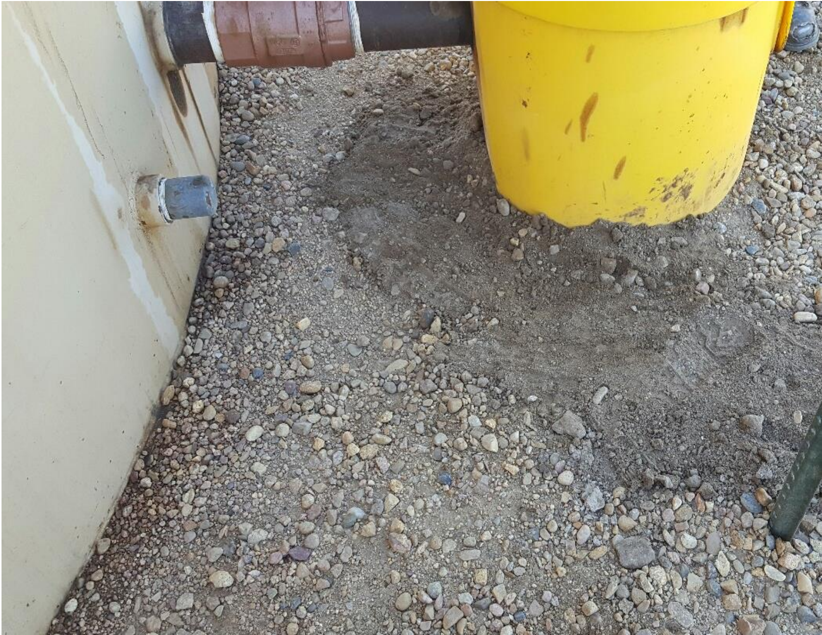
Figure #3 Bull plugs have been installed.
