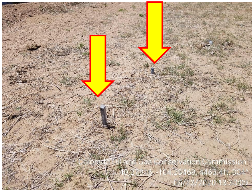
Photo 5 – Unmarked Deadman Anchors by Tank
