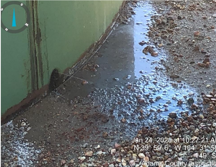
Photo #3 Leak in Condensate tank
