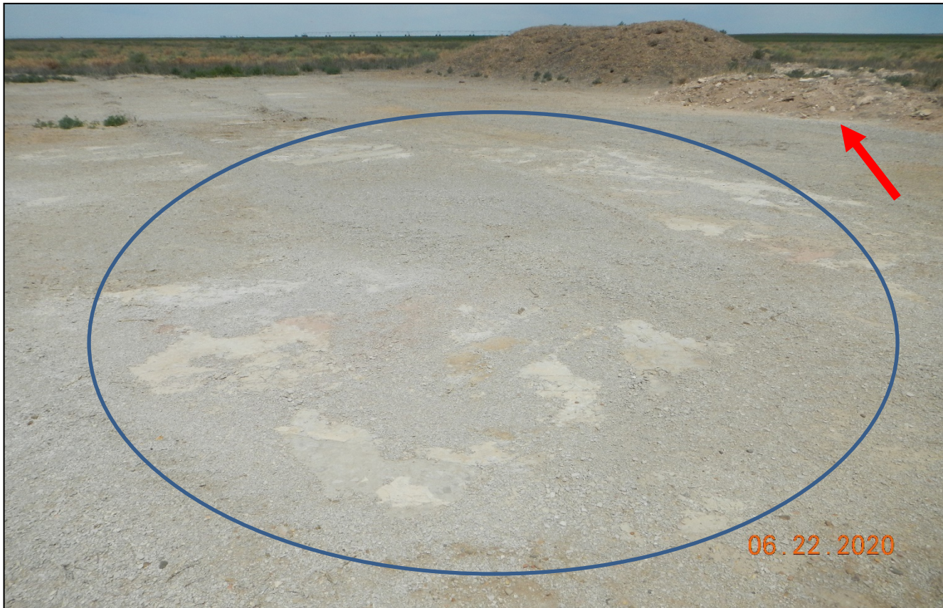
Photo 6. Facing northwest. The piles of soil, gravel/debris remains at the northwest corner of the location (red arrow). There appears to be cement in this area shown in circled area.
