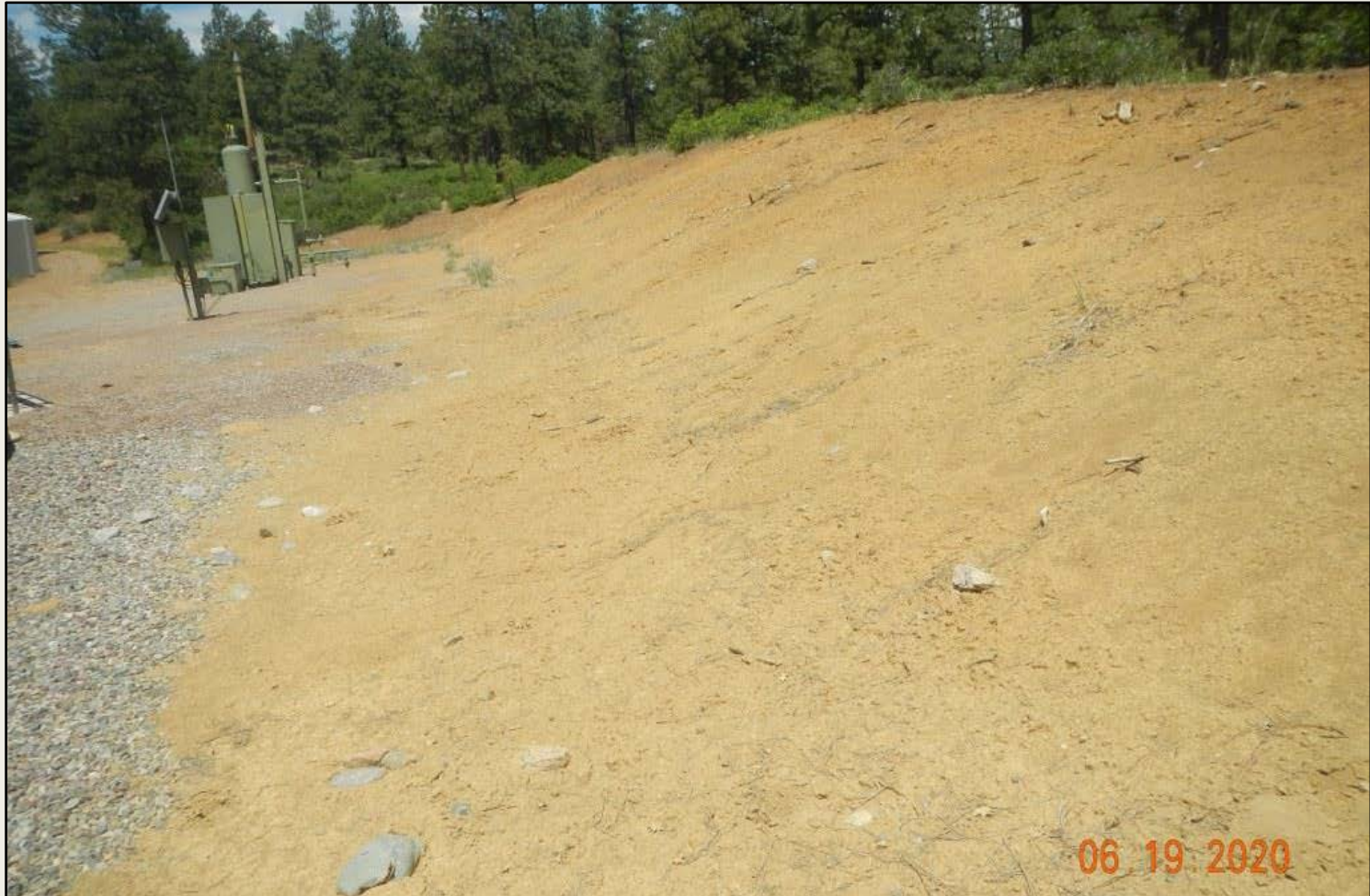
Photo 4. View of the northern cut slope from the northeastern corner facing westward. Stabilization measures are needed on the well pad cut-slope.
