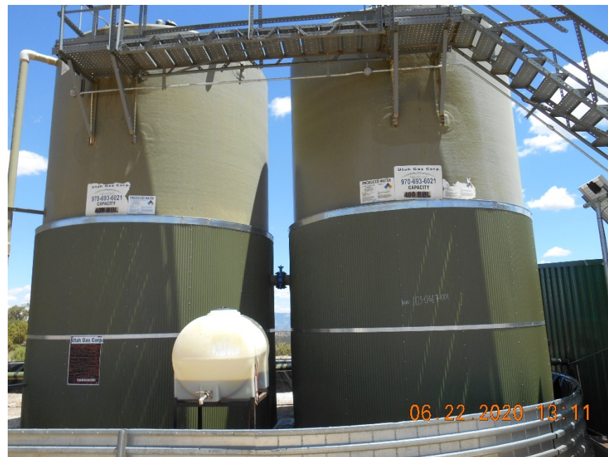
Tank battery and Secondary containment of chemicals
