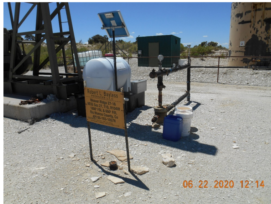
Injection wellhead with sign. 5 gal buckets and container with unknown contents.
