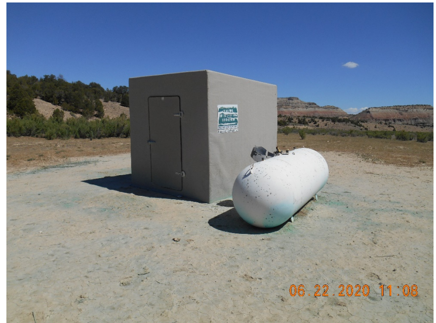
Injection Wellhead housing and propane tank.
