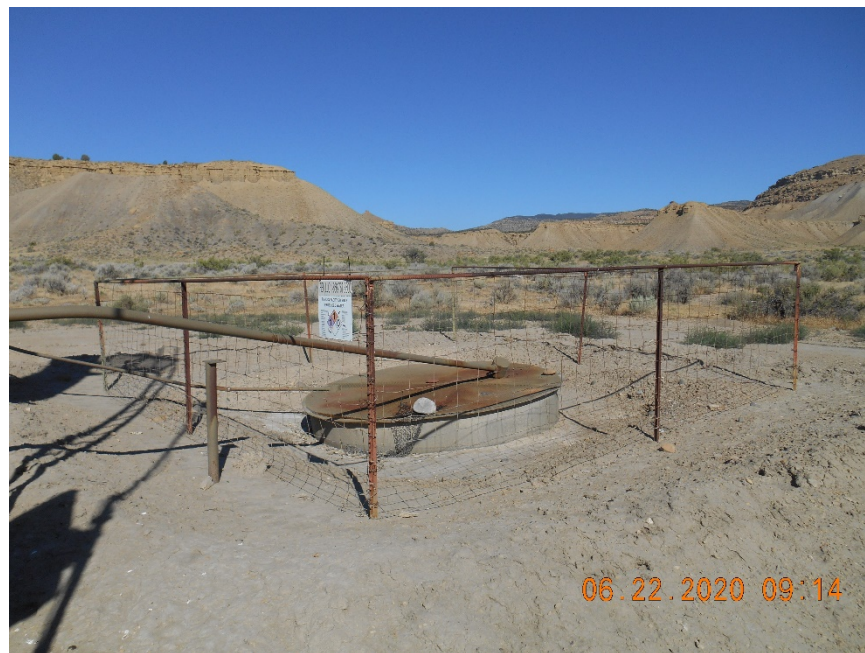
Blowdown tank with fence and sign
