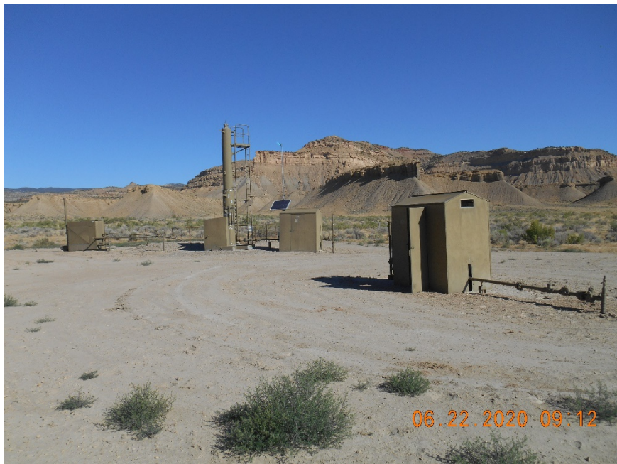
Separator, Dehydrator with blowdown tank, Meter housing
