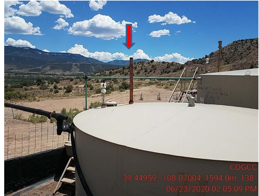
Production tank open to atmosphere
