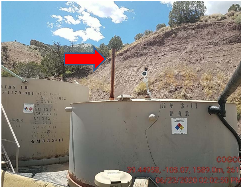
Production tank open to atmosphere
