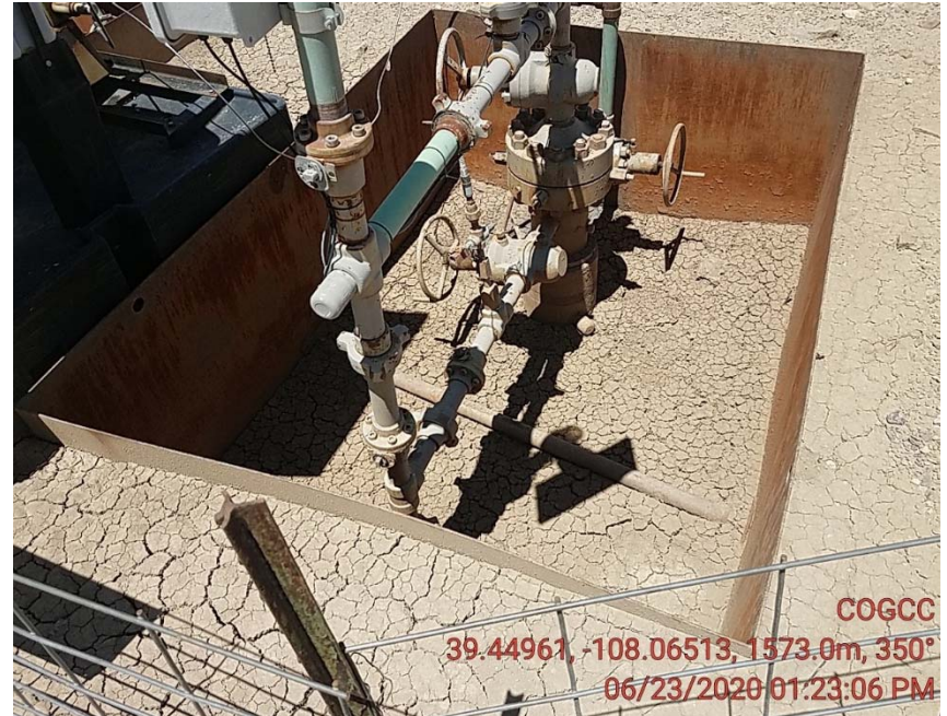
well head cellar with out egress for wildlife
