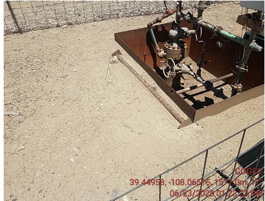
Debris/well head cellar with out egress for wildlife
