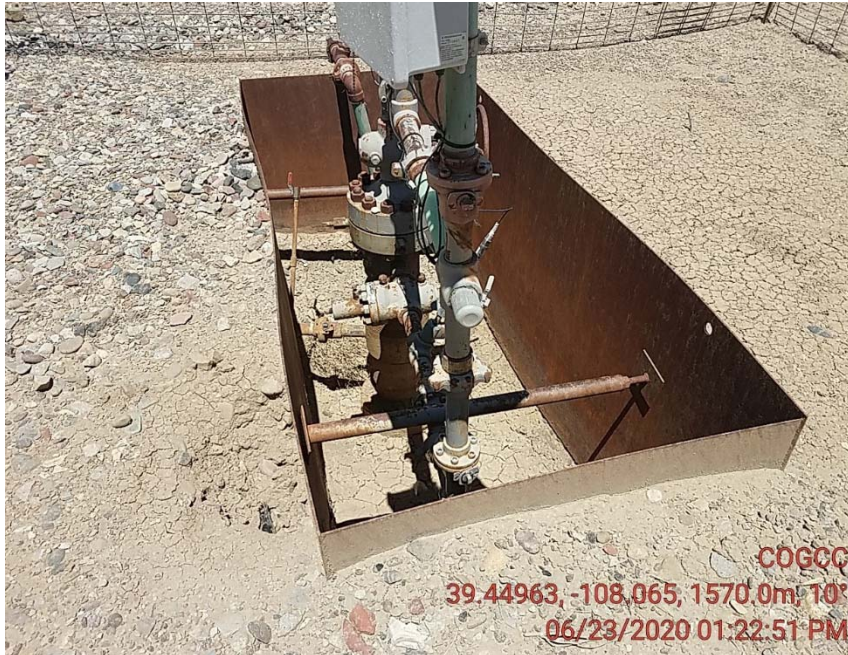
well head cellar with out egress for wildlife
