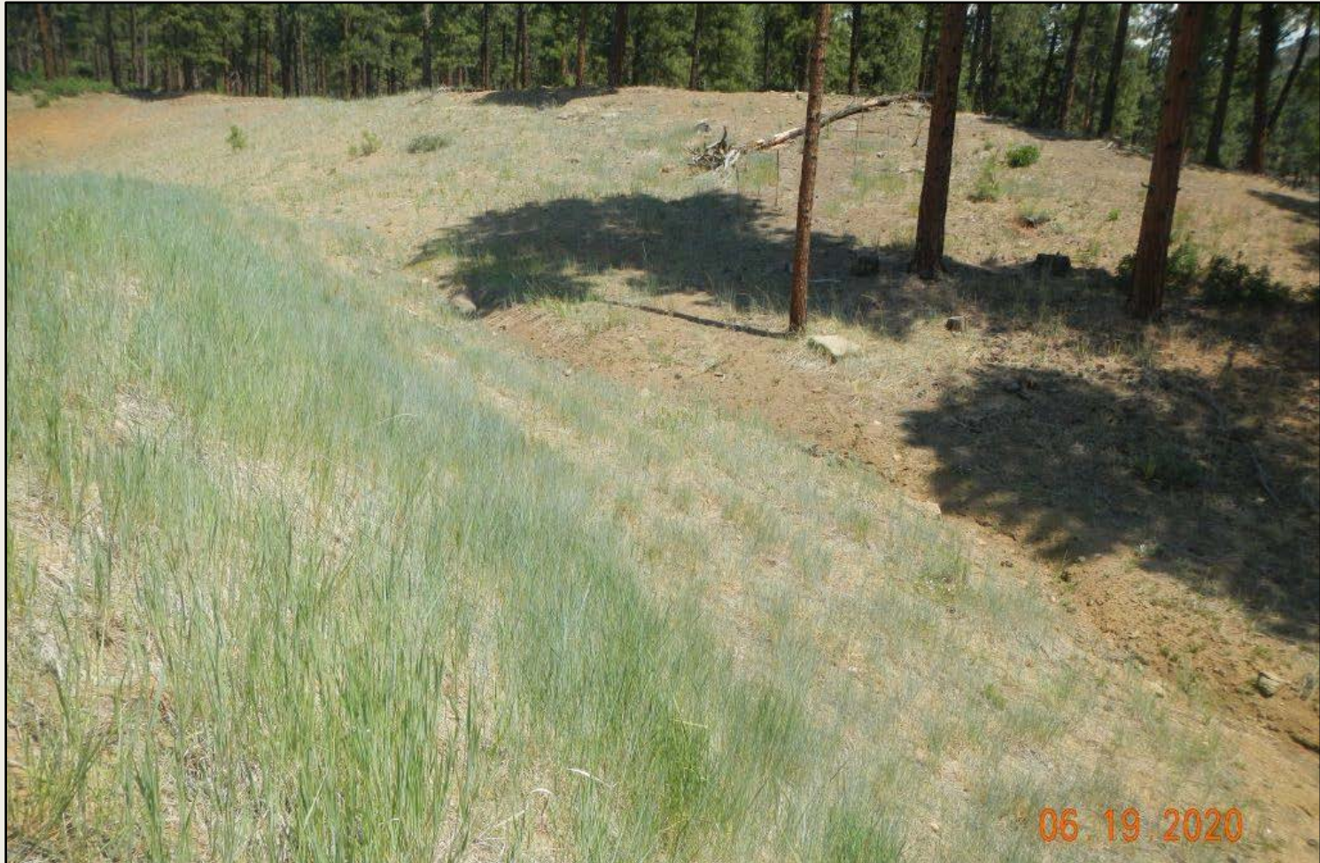
Photo 2. View of the eastern fill slope from the southeastern corner facing westward. Revegetation is progressing, largely with smooth brome and western wheatgrass.
