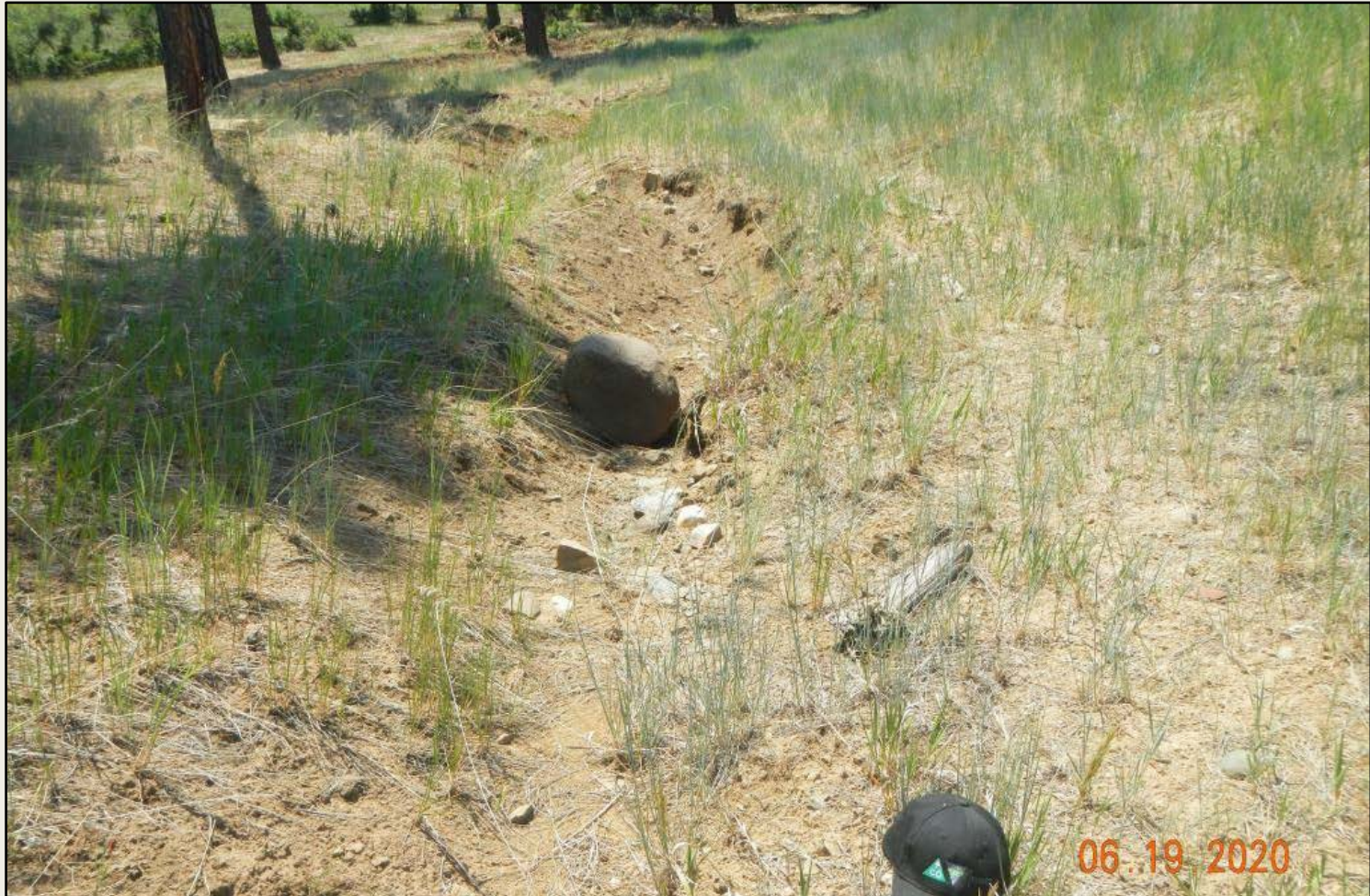
Photo 4. View of erosional channel forming downstream of northeastern diversion, approximately 2 feet wide and 1 foot deep.
