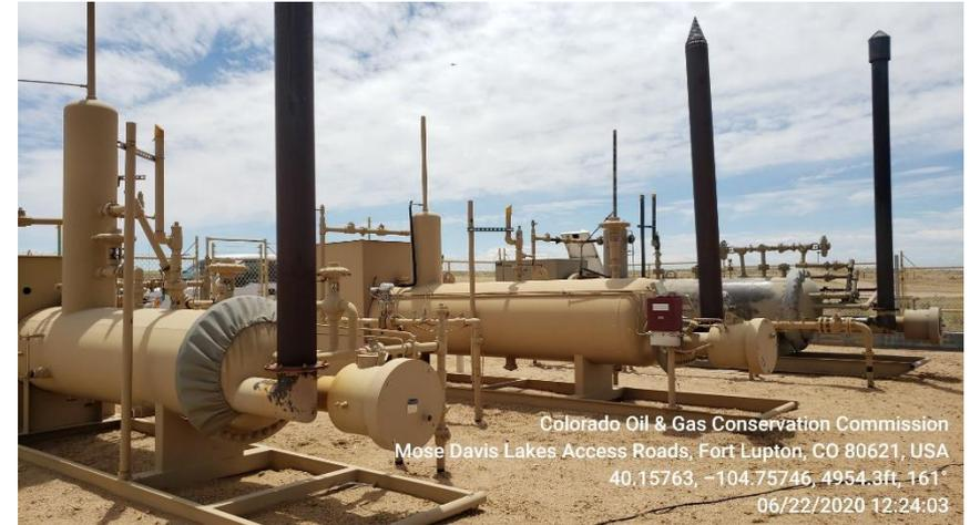
**Photo 5 ECDs, horizontal Heated Separators and Gas meter run**
