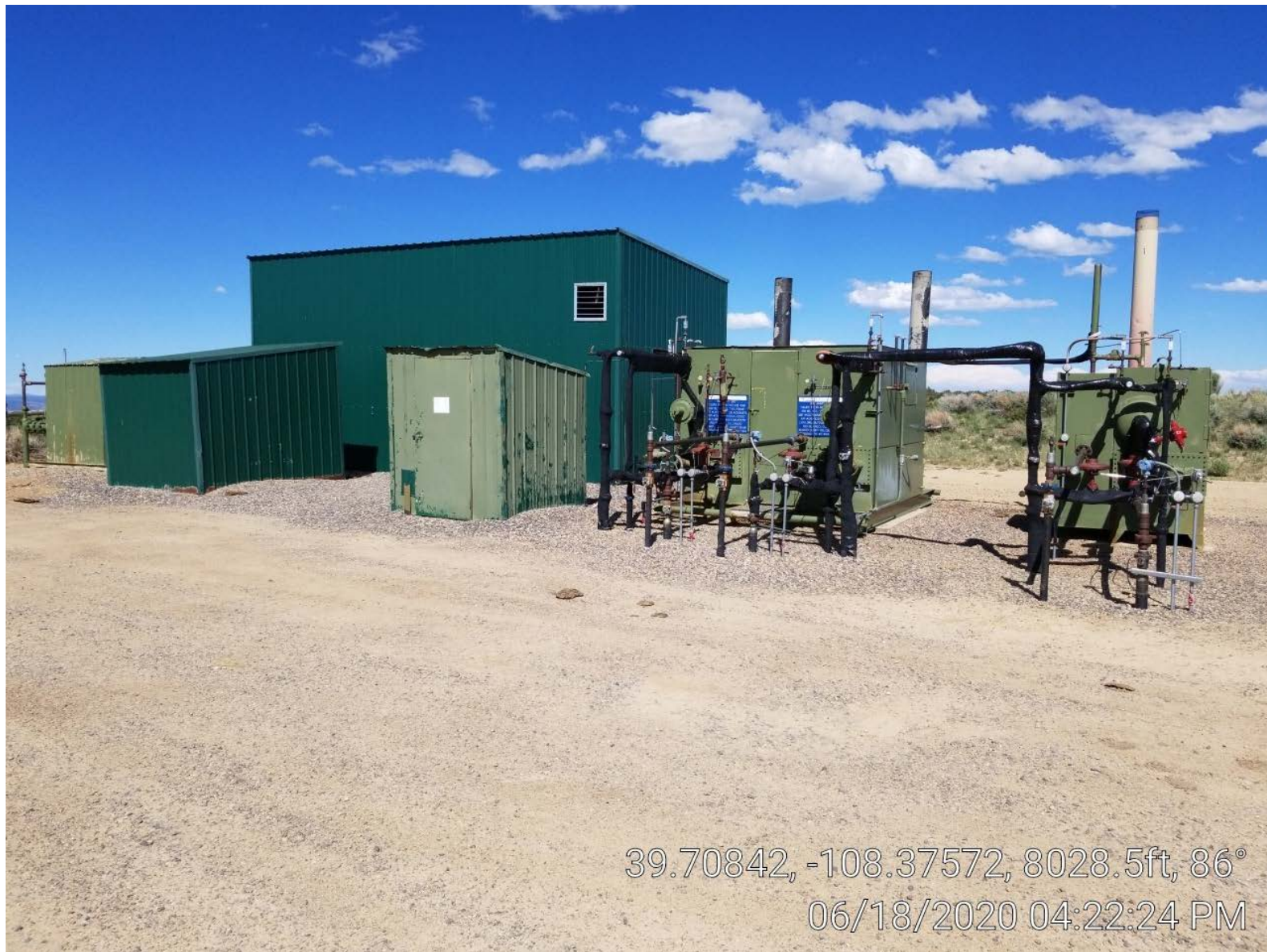
Photo 2. Separators & meter buildings.
