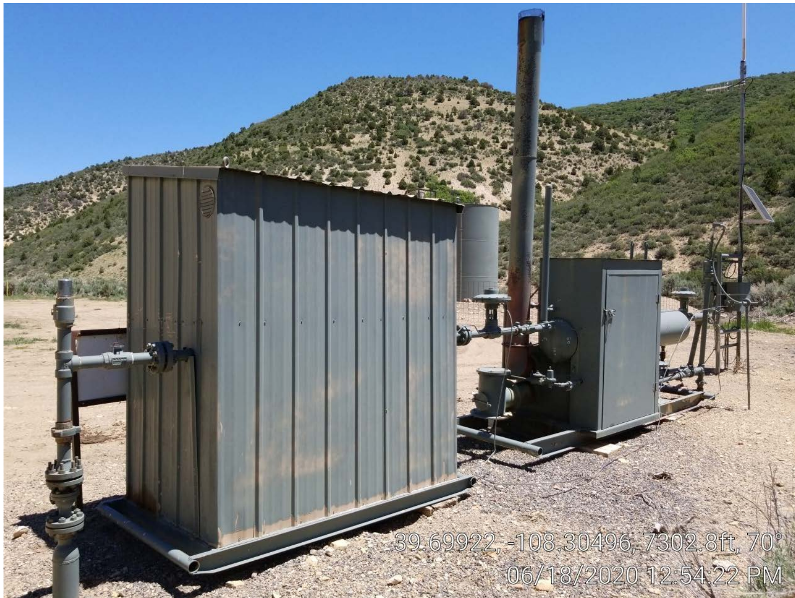
Photo 3. Meter building & separator.
