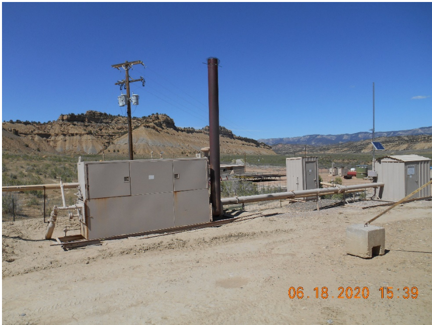
Separator and Meter housing
