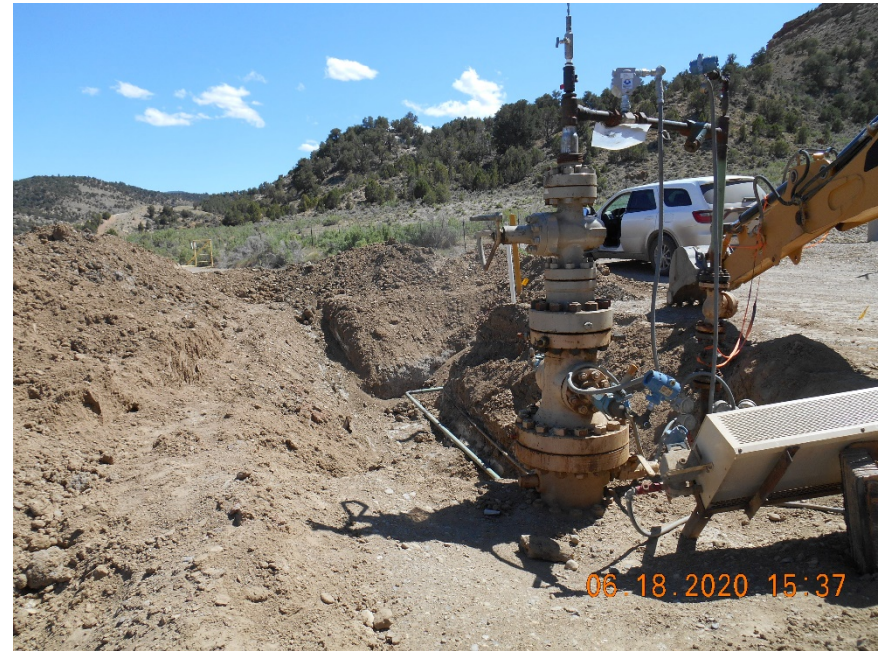
Wellhead with flowline excavated
