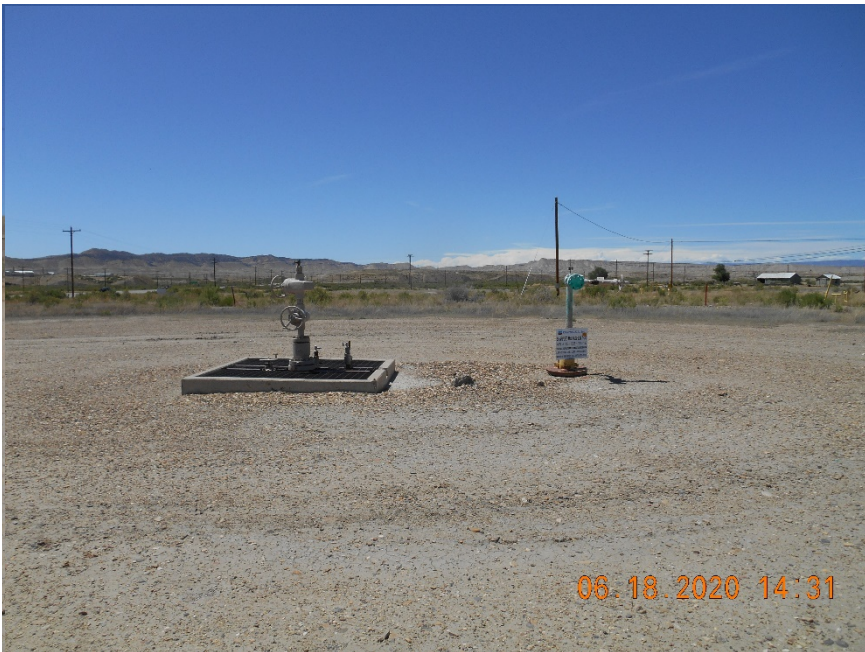
Injection wellhead. Temporarily Abandoned
